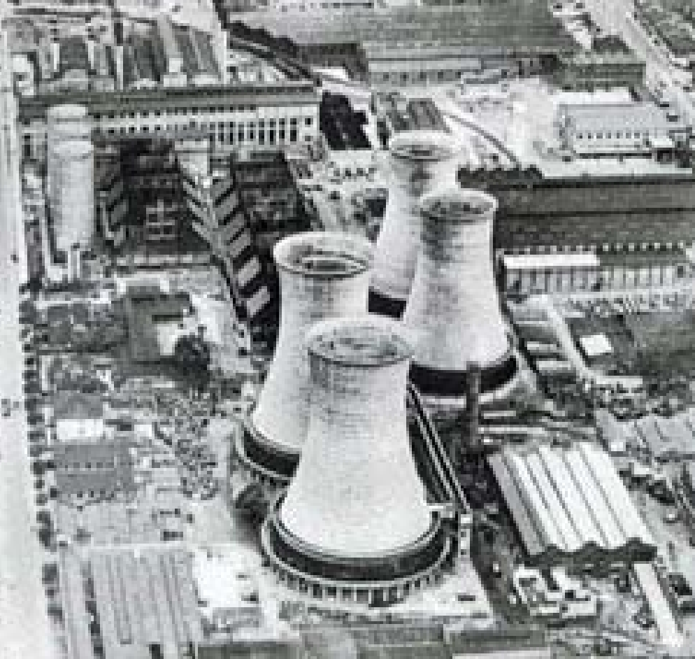
FIG 25. Original Workers' Electricity Compound (No Author Available. n.d.)
