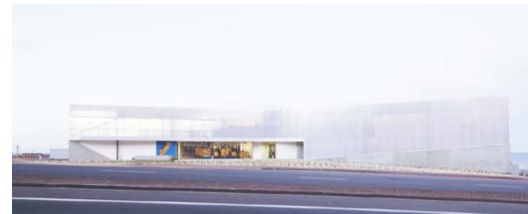
FIG 56. Exterior View of Burnie Makerspace. (Boardman, 2010)
