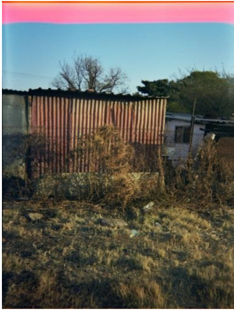
Figure 4 – Upgrading is needed (Kevin)
