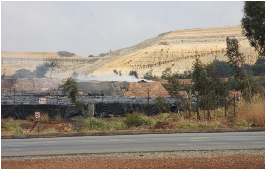
Figure 2-19: Tailings Storage Facility
