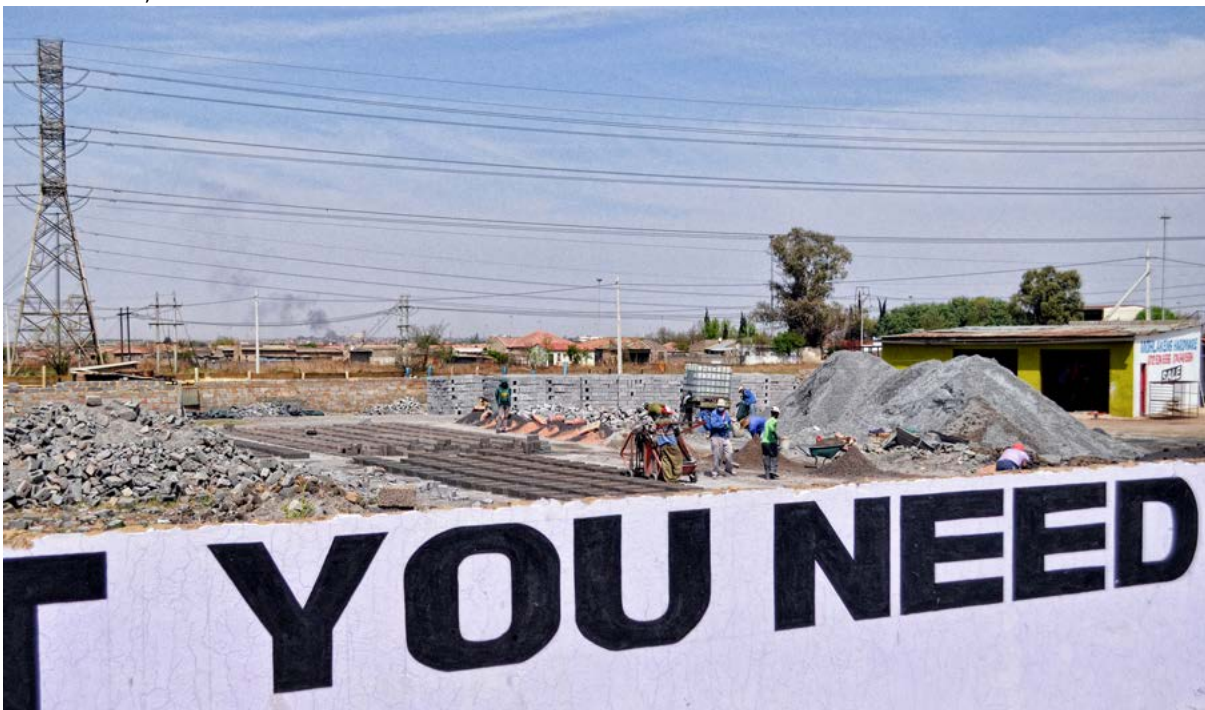
Figure 4.4: Brick-Making and Light Industrial Development - This picture shows an example of one of many brick making light industry located opportunistically on Bierman Road, approximately a kilometre away from Chris Hani Crossing. These are within easy access for people looking to build new houses or renovate existing ones
