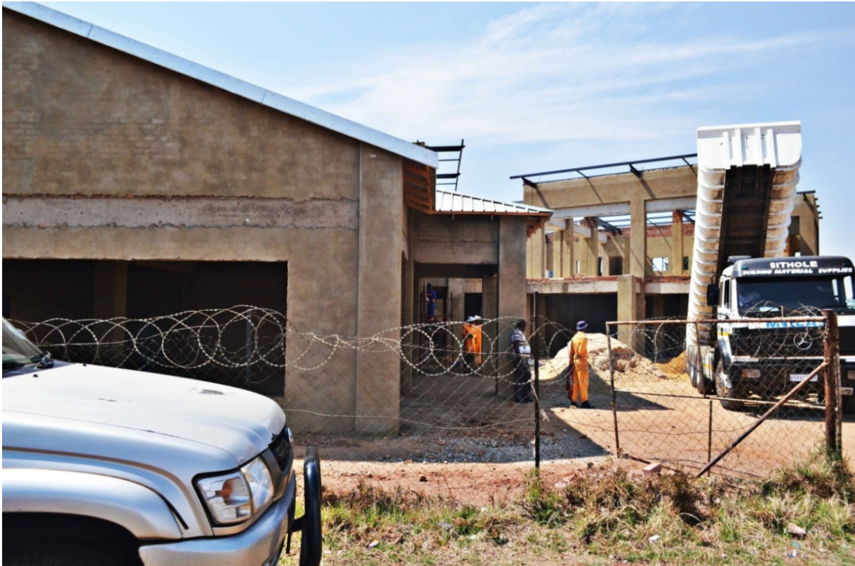
Figure 4.3: New Development - This is a Medical Centre under construction located to the west of the mall which has also capitalised on the availability of increased pedestrian and vehicular traffic. It is the first of its kind in Katlehong and will complement already existing land-uses upon completion.
