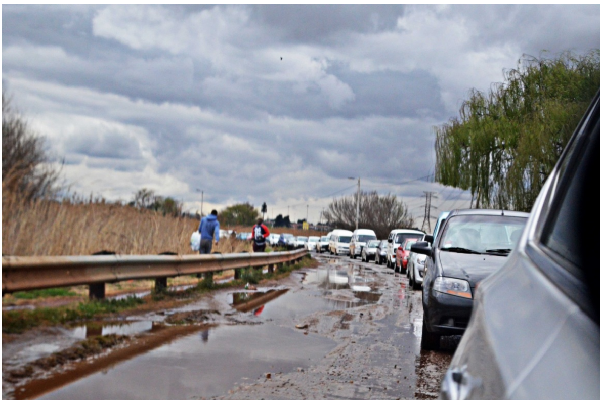
Figure 4.16: Traffic Congestion and Poor Road Infrastructure - This photograph depicts the condition of the road infrastructure and the level of congestion on Bierman Road on a busy weekend during the day.
