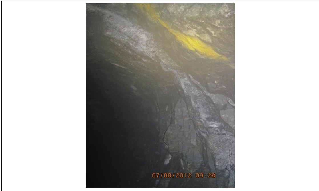
Figure 10.4_2 Face of up dip split before holing showing stress induced curvature over the whole face
