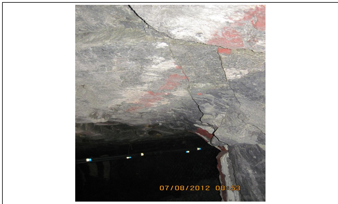
Figure 10.4_1 Edge of pillar in 7N panel, slight curvature at top of pillar and initial spalling, note distinct fractures, on sidewall
