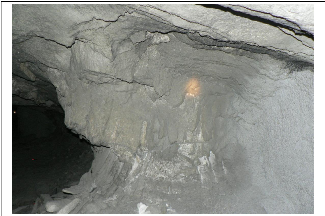
Figure 2.1.8_2 Interaction between pillar and hanging wall on the Merensky Reef - Impala Platinum Mine
