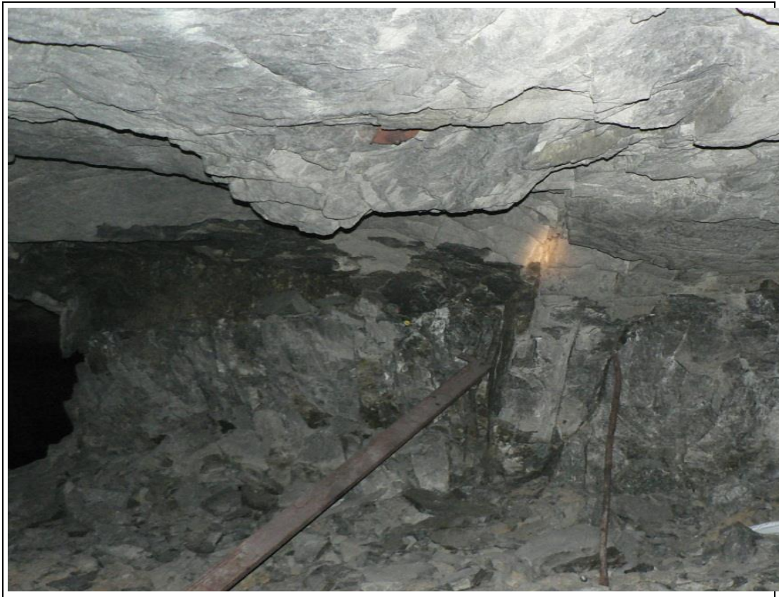
Figure 5.1.3_4 Example of fracturing and estimated GSI value of 80 for a pillar at Impala Platinum Mine.
