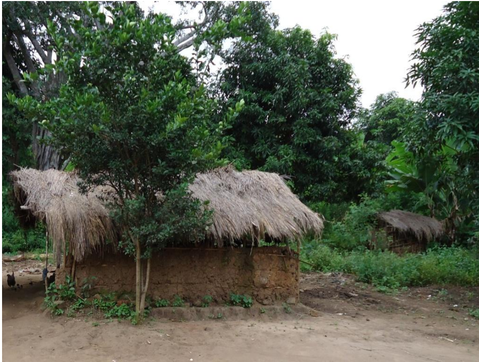
Fig 2.2. Typical shamba house.
