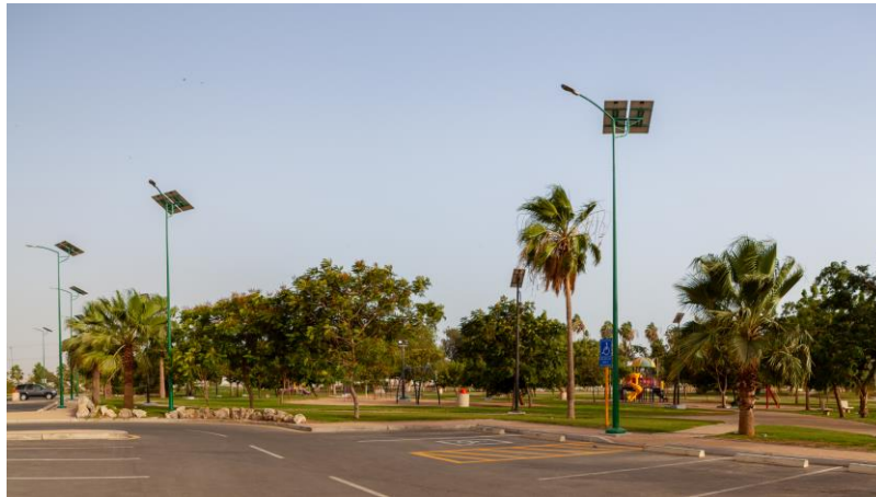
Figure 3.5. A park in Yanbu with solar-powered lamp posts.
