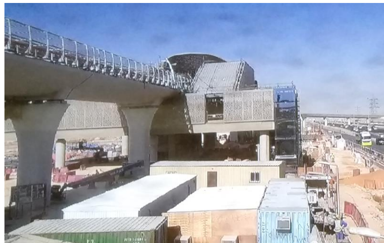
Figure 3.4. Riyadh Metro line and station under construction.
