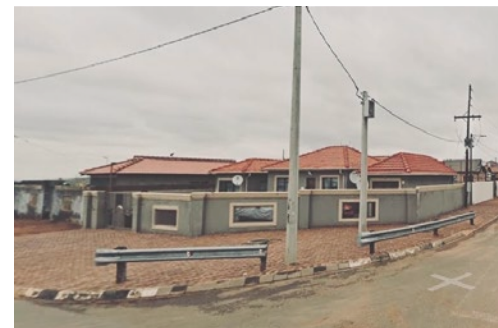
Figure 28 : A housing typology type in Braamfischerville (completely redeveloped RDP), (google maps,2024).
