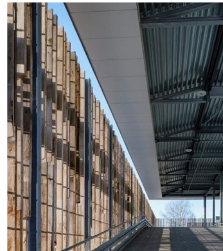
Figure 140 : Facade of Centre constructed using cleared trees from sustainably managed forests, (Modulo,2019).
