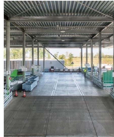
Figure 139 : Repurposed steel roof construction (Anteagroup,2020).
