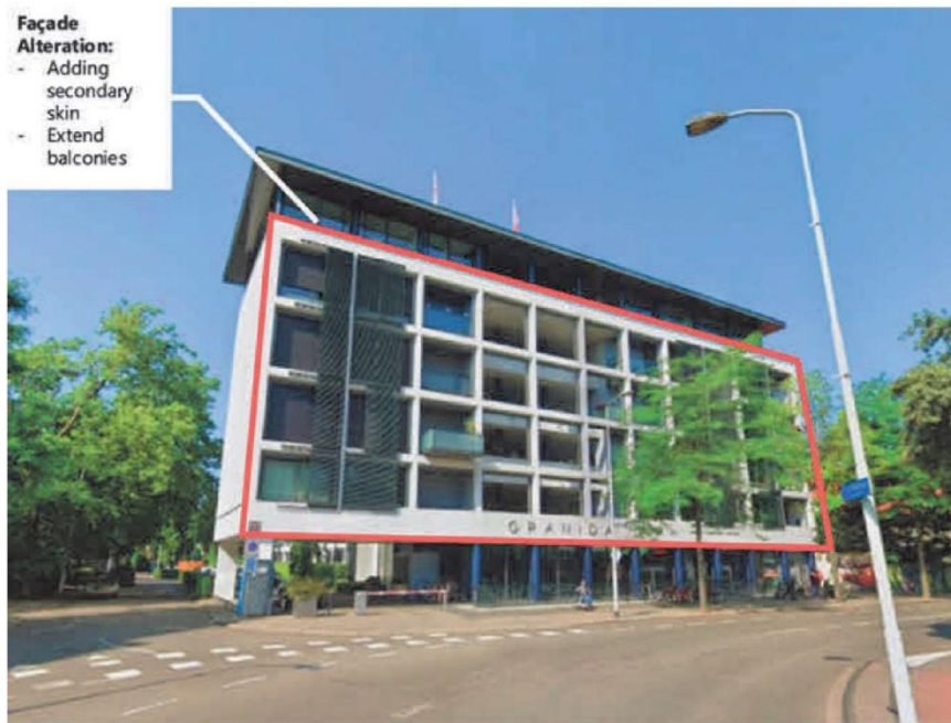
Figure 8 : Granida Building. Mixed use building converted to commercial and luxury apartments in Eindhoven, Netherlands (Pratiwi et al., pp. 439-454).
