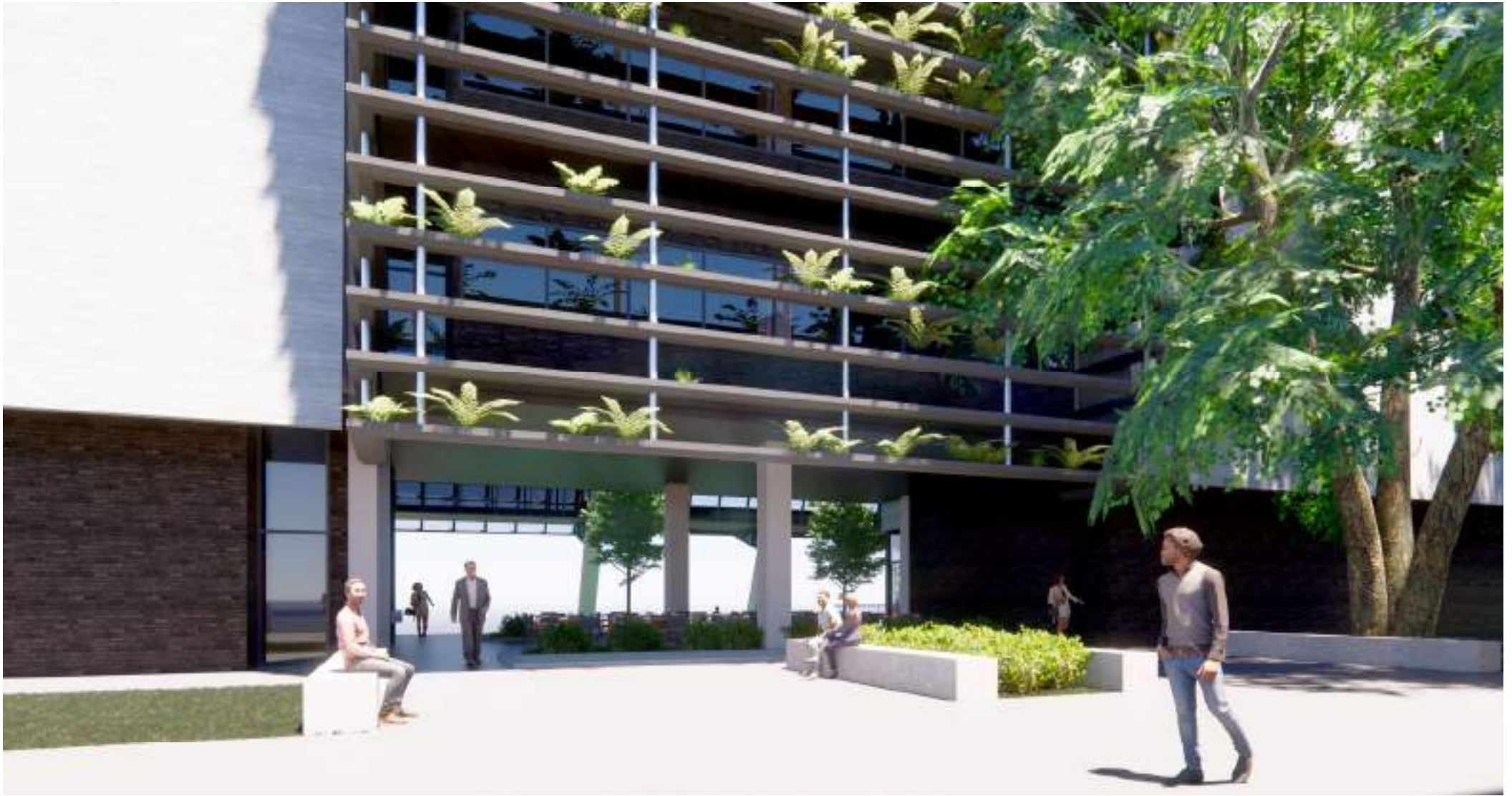
fig. 135. View looking south towards Cafe seating and central atrium space (Author, 2020)
