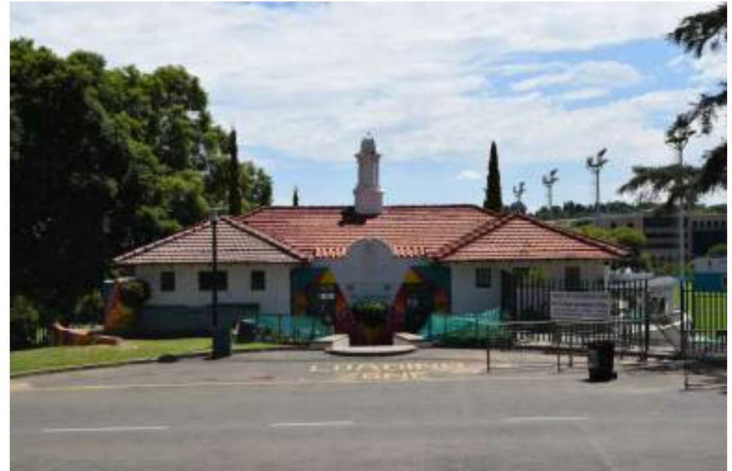
fig. 36. The Sanctuary Building, the home of the Food Sovereignty Centre, Wits East Campus (Author, 2020)
