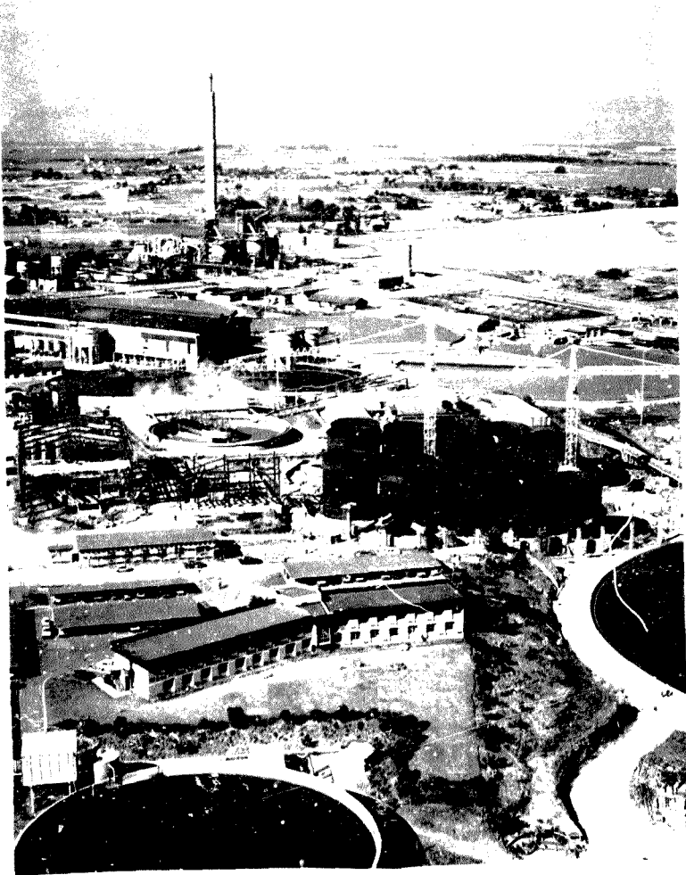
Figure 1.1 The Ergo Division plant in May 1984 with the carbon-in-leach plant being built in the foreground. The flotation plant stands between the thickeners with the gold, uranium and acid plants in the background.
