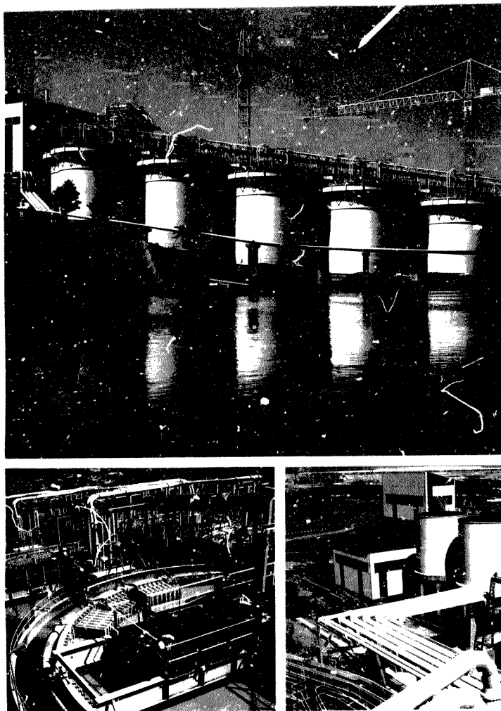
Figure 6.1 The Ergo Division carbon-in-leach plant in February 1985. The leaching and carbon contact tanks are shown in the upper and lower left pictures. The carbon elution building is on the left in the upper picture and the carbon-handling plant is featured at lower right.
