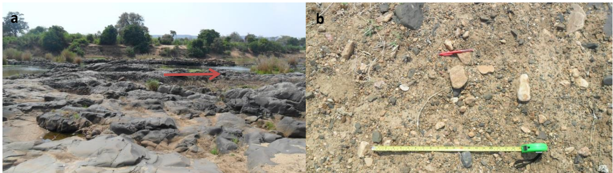
Fig. 5.18: (a) Site 12 characterised by bedrock outcrops. (b) A 20/20 cm square indicating the cobbles present in this reach.
