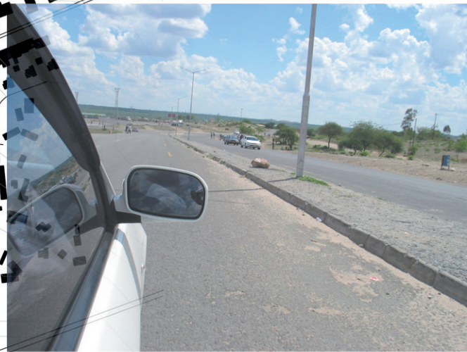
Fig 2.5.2. The traffic circle approaching the border.
