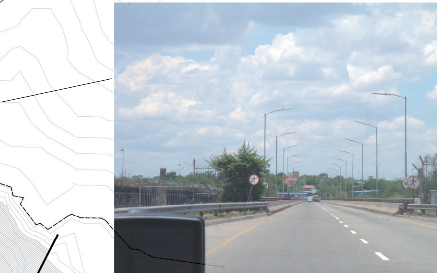
Fig 2.5.4. Entrance to the vehicular bridge
