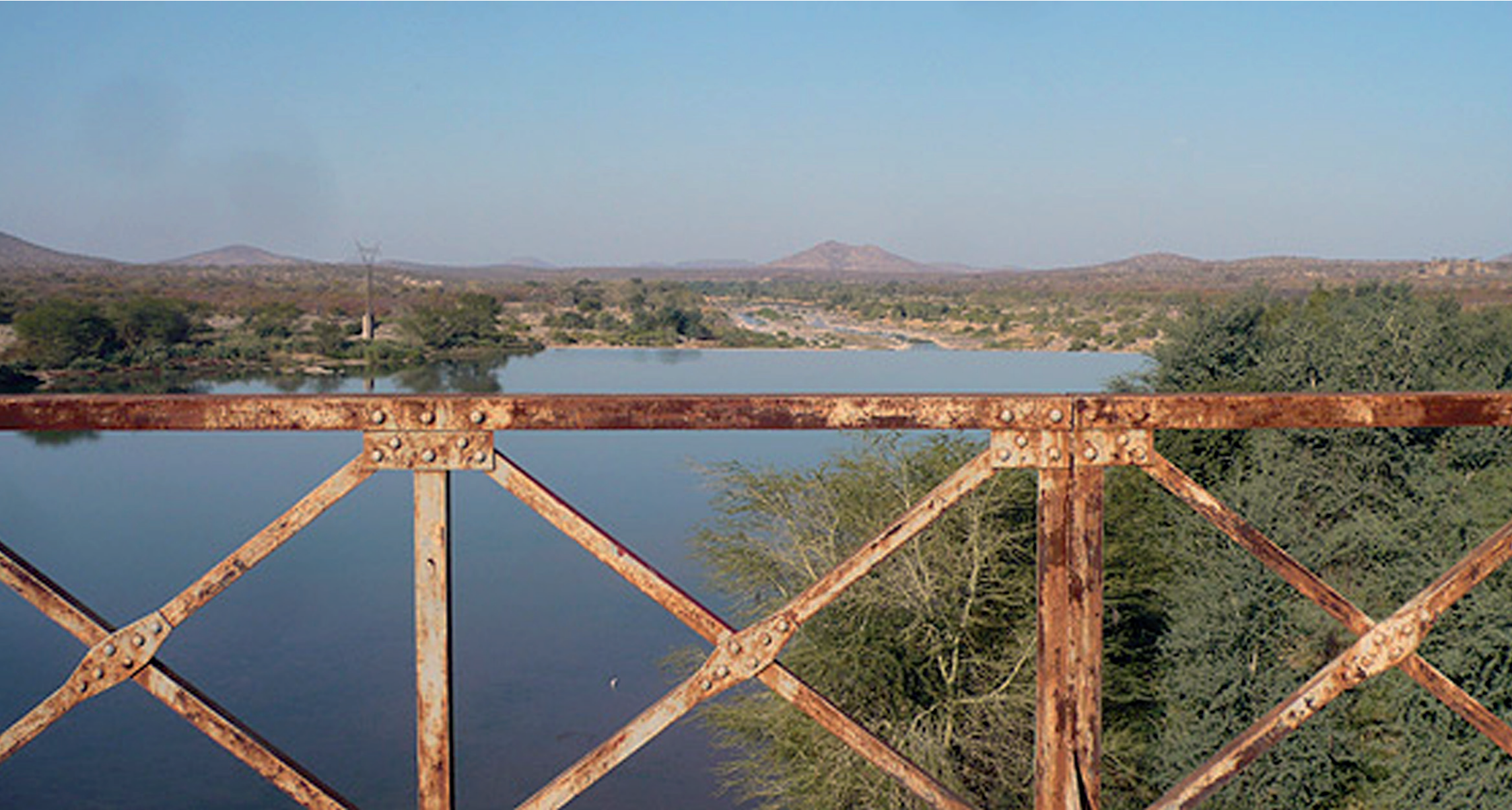
Fig. 3.2.15. View from the Rail/Pedestrian Bridge towards the dam wall
