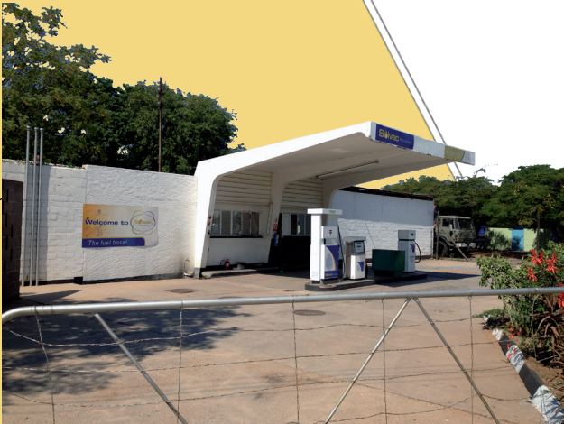
Fig 2.3.11. A Service Station adjacent to the Peter's Motel
