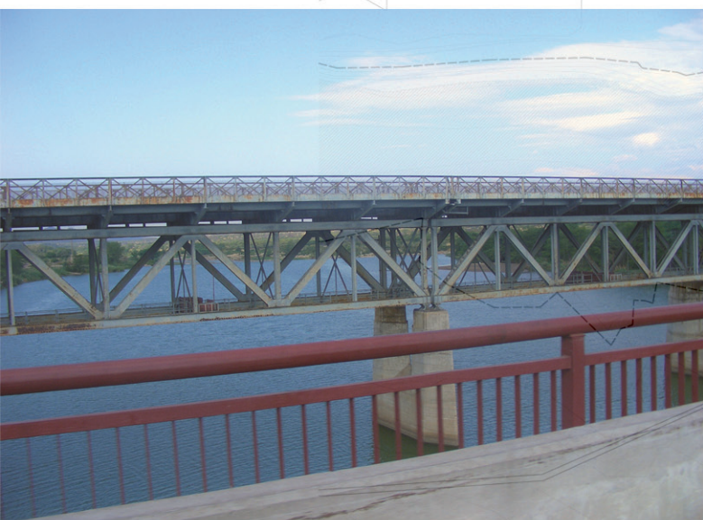
Fig 2.5.5. The Alfred Beit bridge from the vehicular bridge
