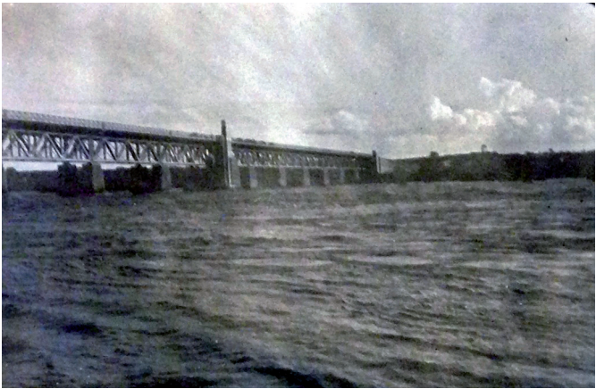
Fig 2.2.3. The Rail bridge shortly after completion in 1929.
