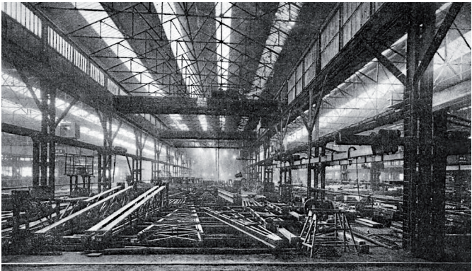
Fig 2.2.6. The Dorman, Long and Co. Bridge and Constructional works Middlesbrough Fabricating Shop where the railway bridge would have been assembled before it was shipped to the its present day location
