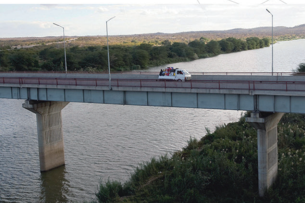
Fig 2.5.6. The vehicular bridge
