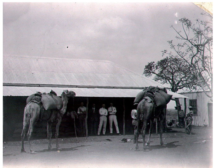
Fig 2.3.5. The first Police Station in Musina. Camels were used for transport
