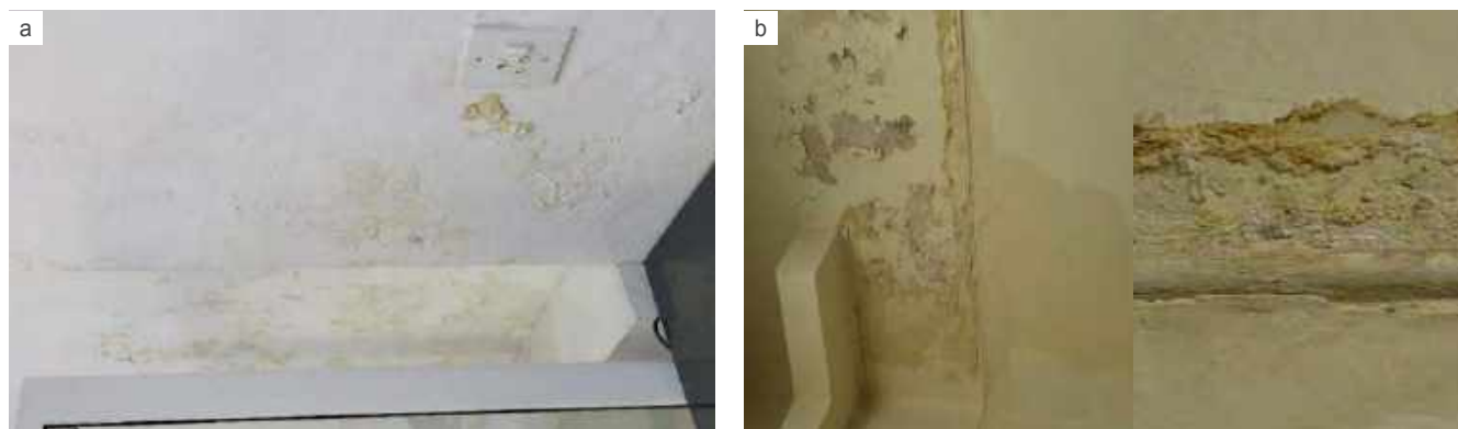
Figure 1: Photographs of visible mould on wall surfaces of areas investigated: (a) clinic room wall with mould growth and (b) X-ray file data storage room.
