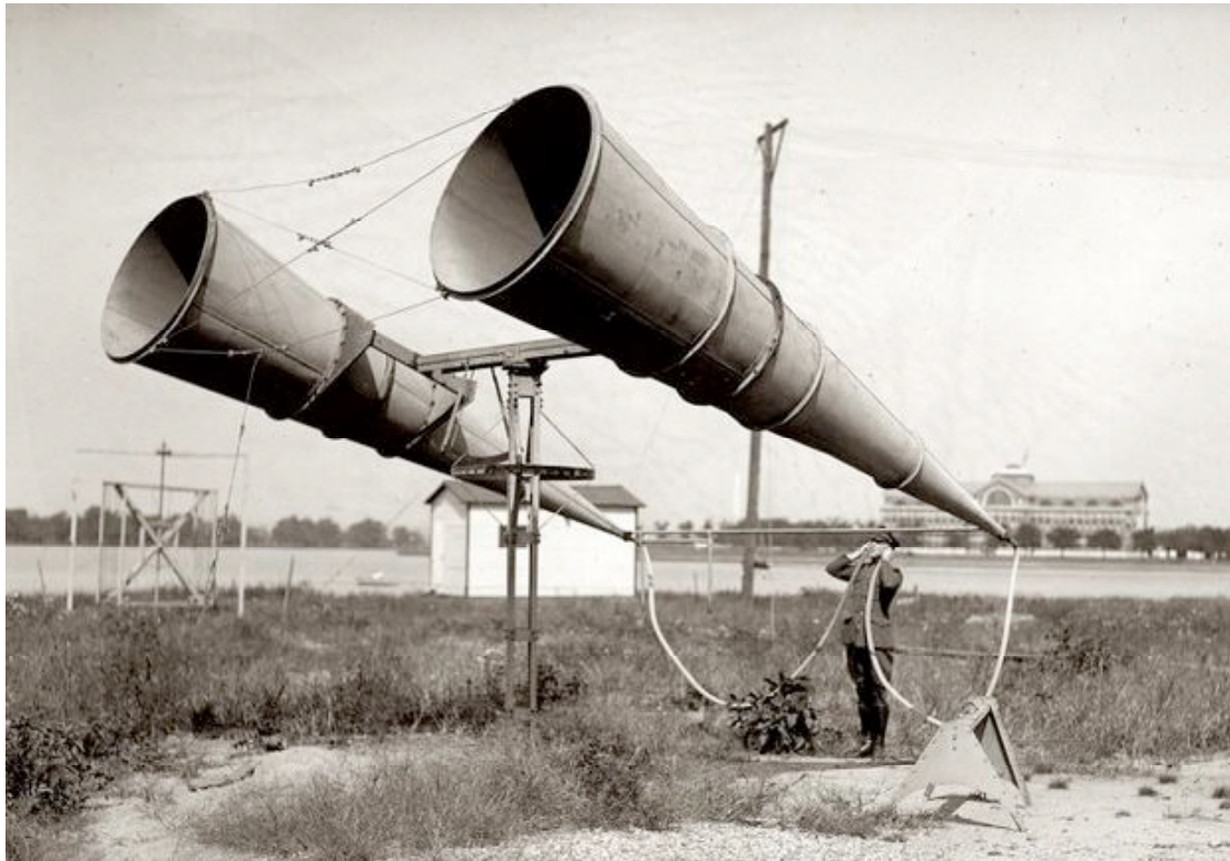
1. A two-horn location system at Bolling Field, U.S.A. (1921)
