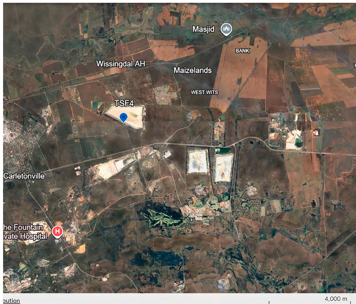
Fig. 1. Google Earth imagery of the tailings (TSF 4), the study site.
