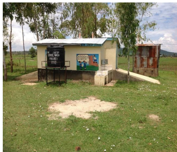
Figure 4 Raised latrines in School C, a GoK/UNICEF project
