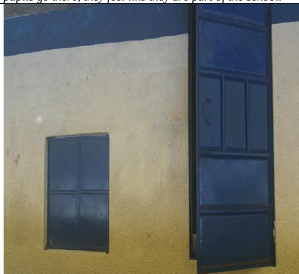
Figure 3 Permanent door structures in School E
