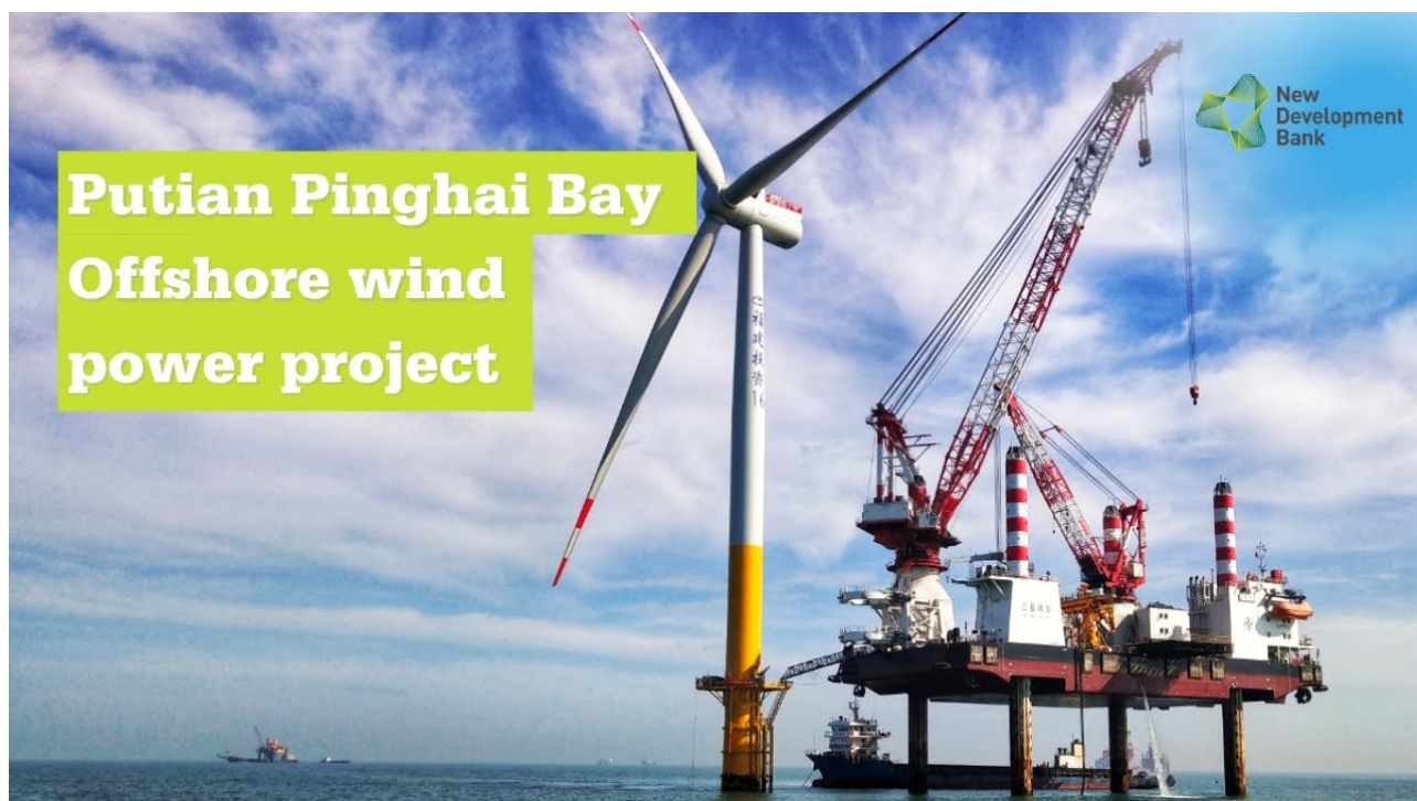
Figure 3.7 - Construction of the NDB co-financed wind power plants in Pinghai Bay, Fujian
