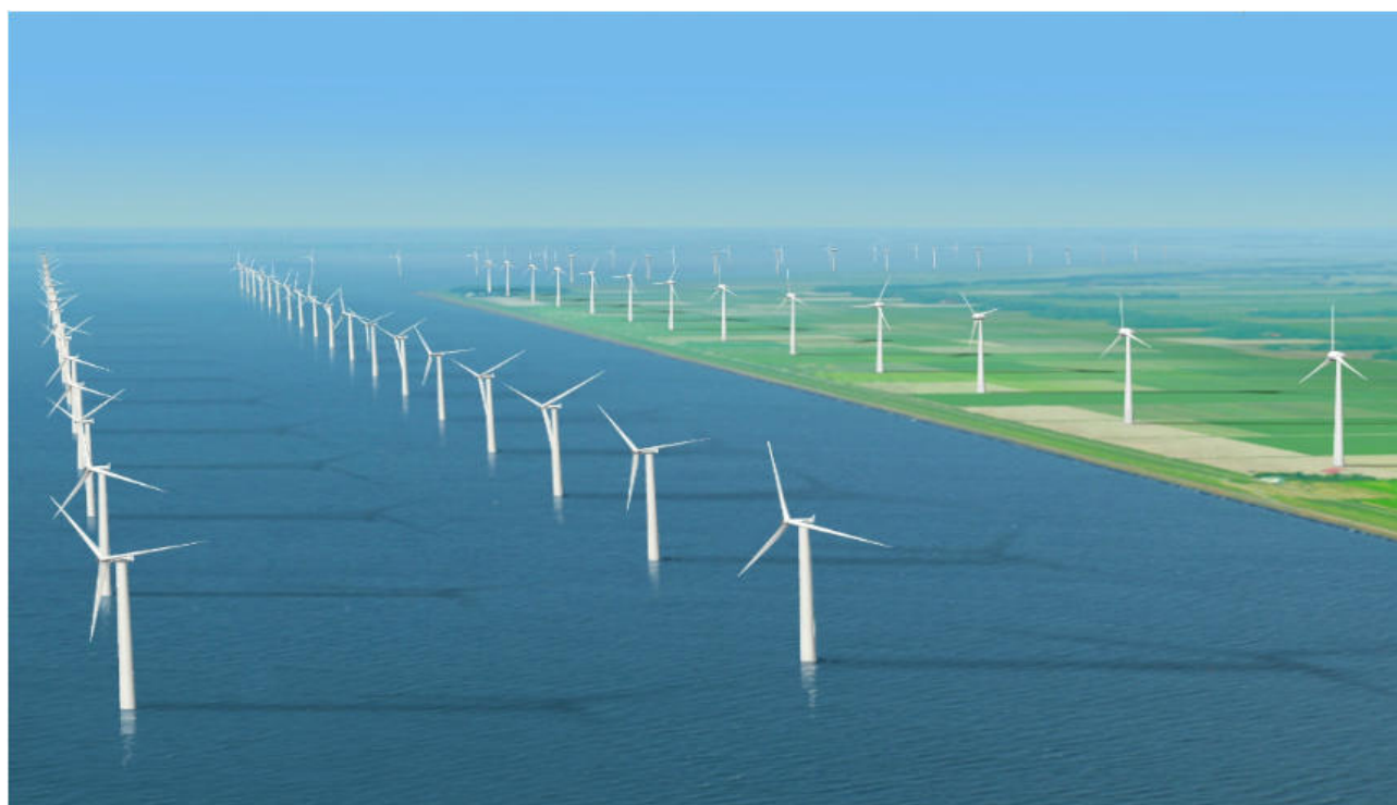
Figure 3.8- The NDB co-financed wind power plants in Pinghai Bay, Fujian
