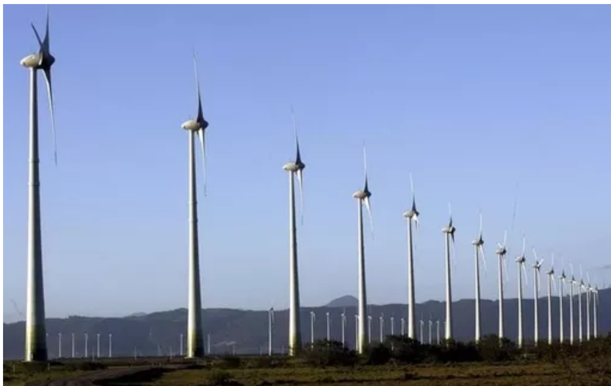
Figure 3.2 - The NDB co-financed wind power plants in Araripe, Ceará
