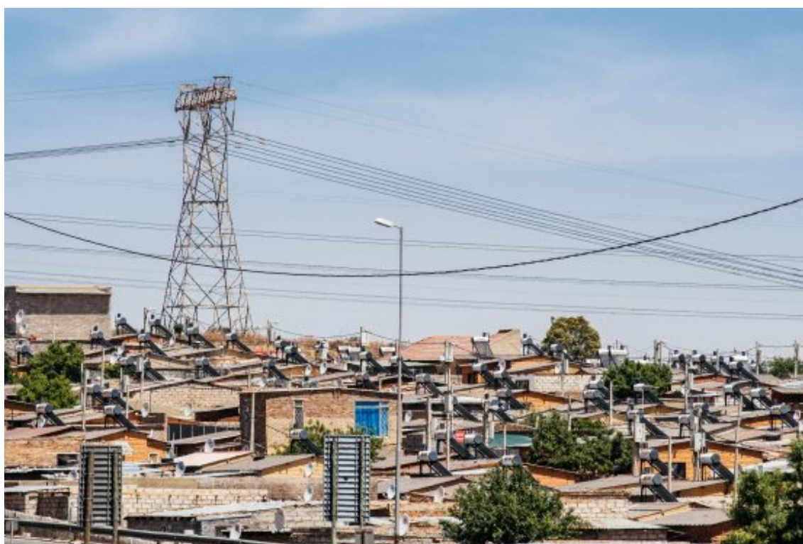
Figure 3.10 - Eskom's electricity grid network in Soweto, Gauteng
