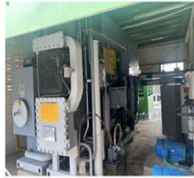
Figure 4. Series double-effect absorption cooling system. (a) Adapted from [32], (b) photo taken from UTB.
