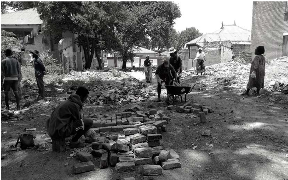
Figure 16: Co-production, the beginning of the construction process in Bertrams (Author, 2020)
