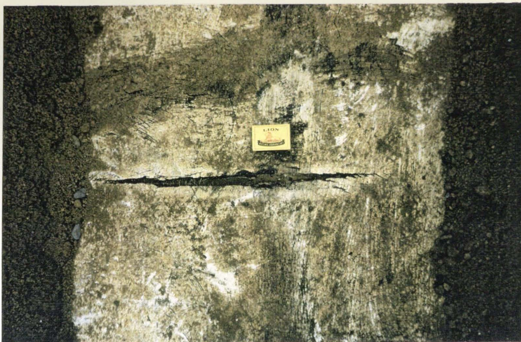
PLATE 12 A tension crack in the bitumen insulation on the pipe.
