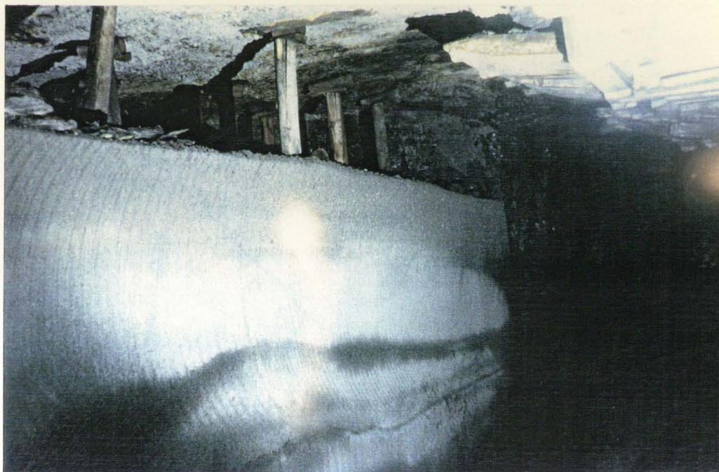
PLATE 4 The fill material which was placed in the roads before mining to stabilize the area, shown here during the mining operation.
