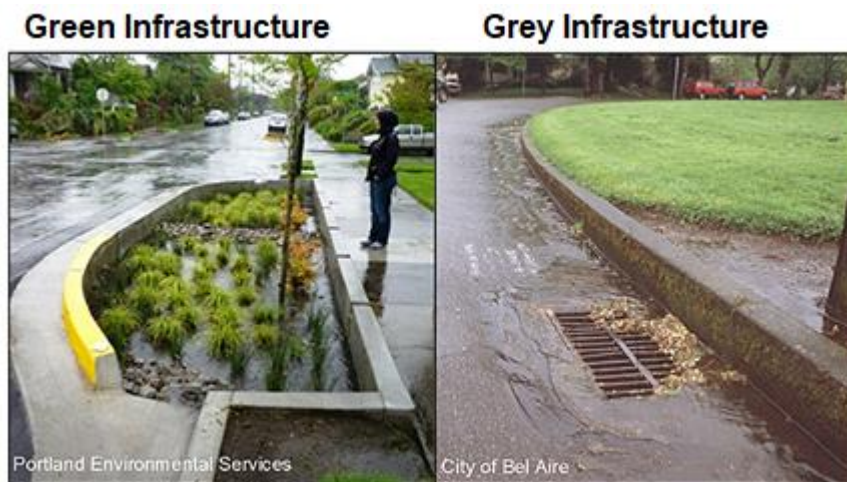
Figure 2.2 - Green vs Grey Infrastructure (Lagasse, 2015)
