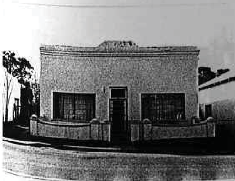
325. Erf 130; 11 West Church Street.
