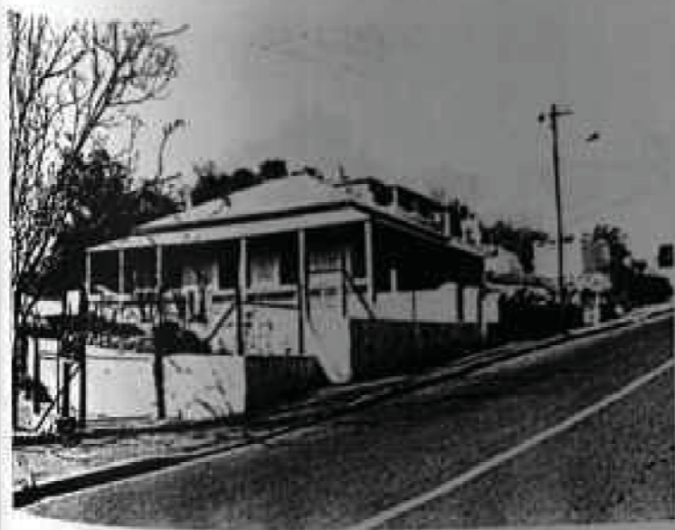
8. Erf 134: ? West Church Street.
