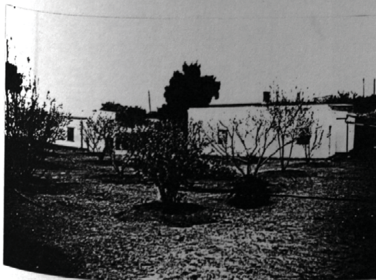
371. Erf 21: Outbuilding of 1 Loch Street.
