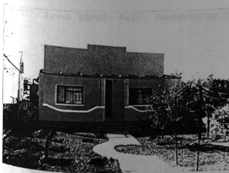
376. Erven 58, 59 & 57: 21 Ventershoek Street.
