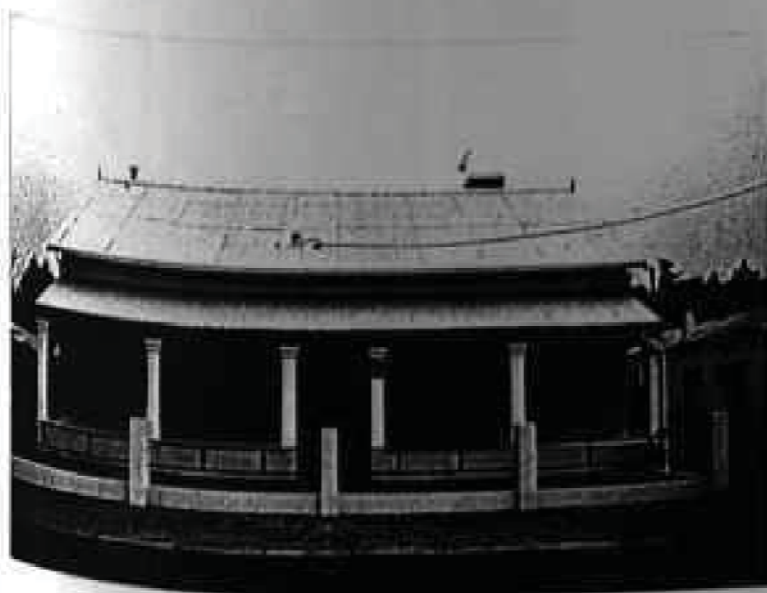
358. Erf 37: 21 West Church Street.
