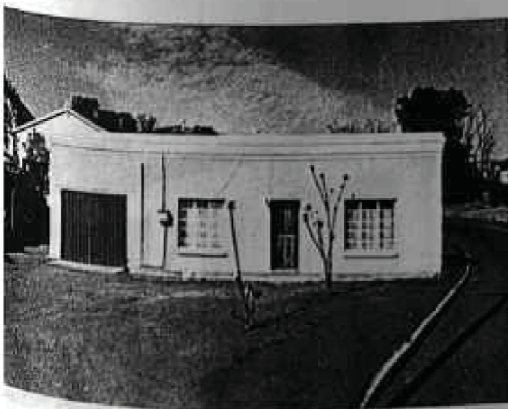
331. Erf 137: ? West Church Street.
