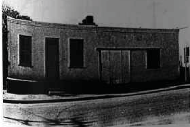
308. Erf 131: ? West Church Street.
