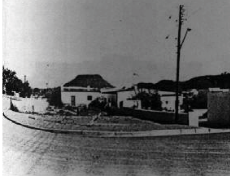
374. Erf 54: Back of 25 Ventershoek Street.
