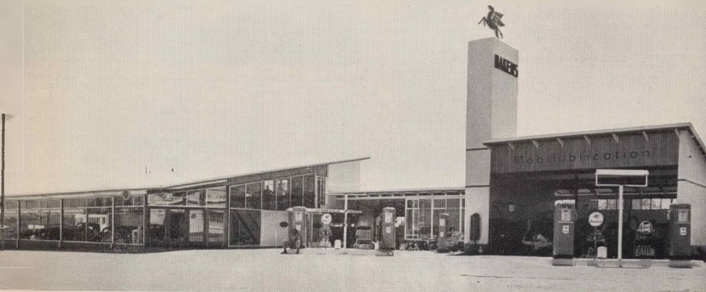
View of garage from south-east.
