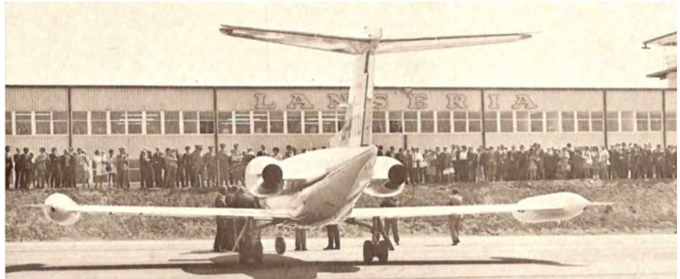
△ Figure 3.11 View of Lanseria Airport terminal in 1975 (Lanseria International Airport, 2010 : Online)
