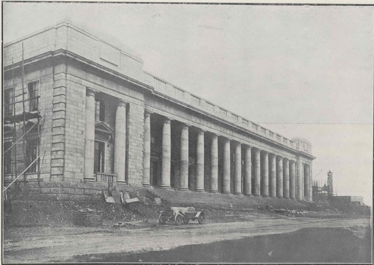
Chemistry and Physics Block. University of the Witwatersrand. North Front to Campus.
