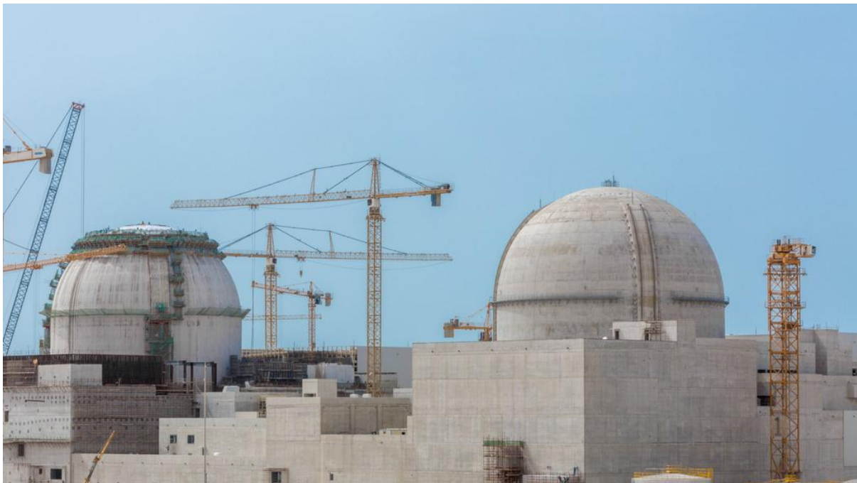
Figure 2.1: A United Arab Emirates NPP under construction (source: Scmp.com 2017)
