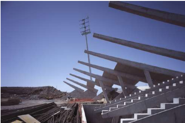
Figure 5.16 (above): Concrete portal frames are the main structure
