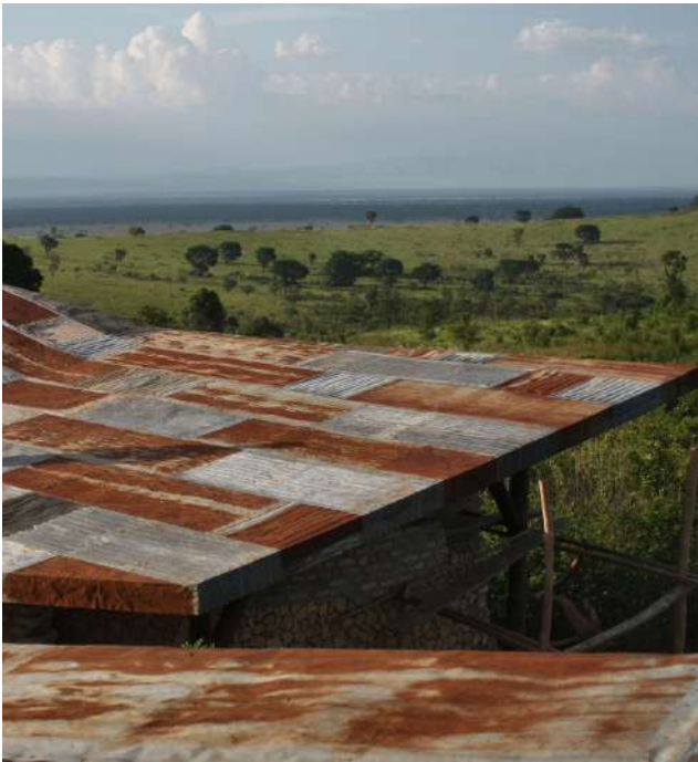
Figure 5.2: Use of discarded rusty steel for roofing Image source: https://archello.com/project/kyambura-gorge-lodge
