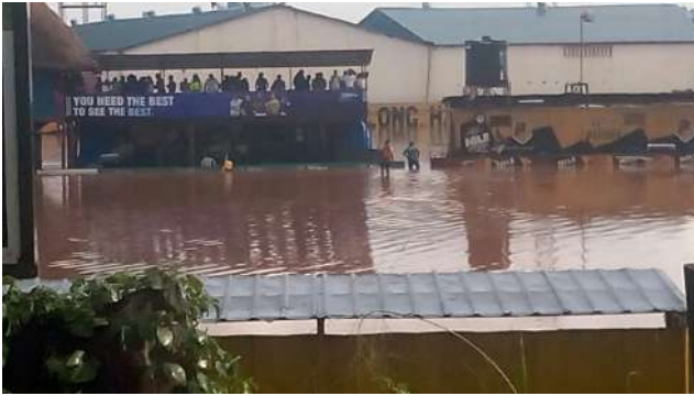
Figure 4.23: The extent to which the rugby grounds flood after heavy rains
