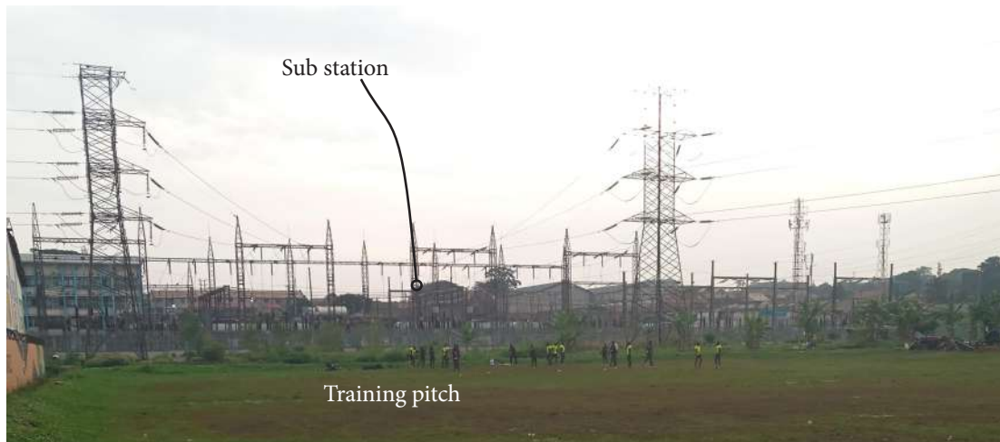
Figure 4.29: The power station on the background relative to the training pitch (Author's photograph)
