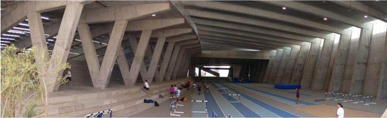
Figure 5.16 (above): Concrete portal frames are the main structure
