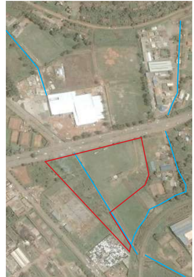
Figure 4.16: Lugogo junction in 2004; At the start of the development of Lugogo Shopping mall, some of the green areas were encroached upon; an underground drainage channel was constructed in order for the construction of the shopping mall to start.
