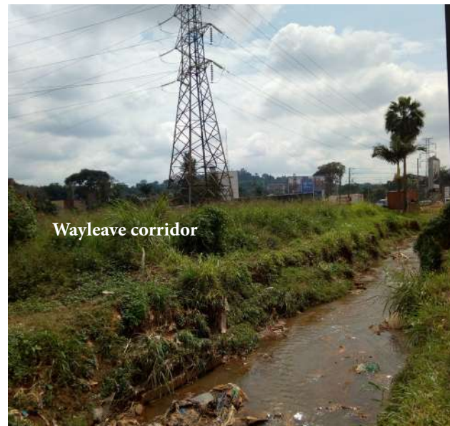
Figure 4.41: Drainage channel bordering the wayleave corridor and rugby pitch (Author's image)
