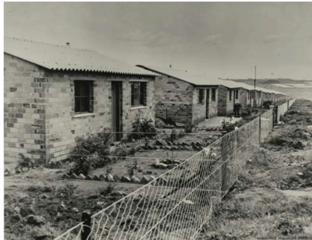
Figure 4.3 A street view of Orlando housing (Foster, 2012: 51).
