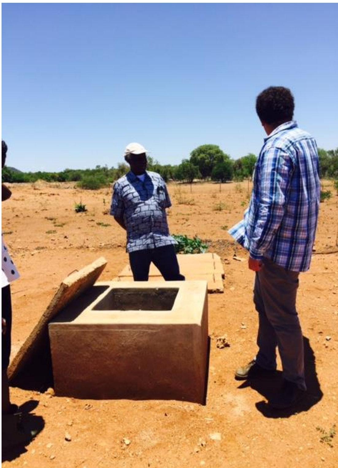
Picture 7: A concrete underground biogas digester in Gawula
