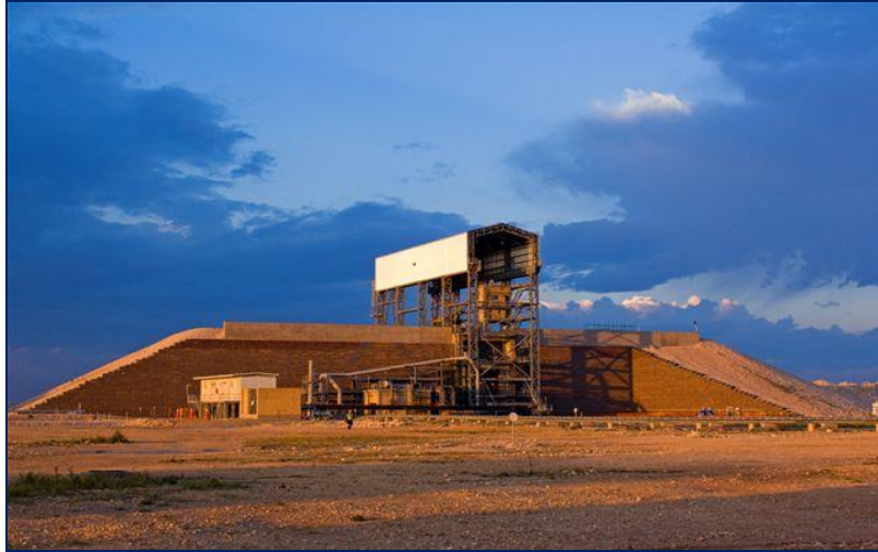
Figure 5.12. Kolomela primary crusher
