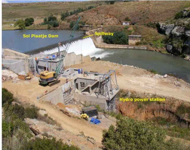
Figure 21: The Sol Plaatje Hydropower Project: construction underway
