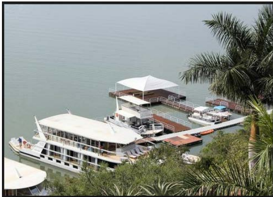
Figure 2: A Boathouse on the Jozini Dam
