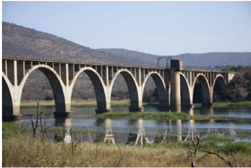
Figure 8: Pongola River Railway Crossing Water Level in September 2009.
