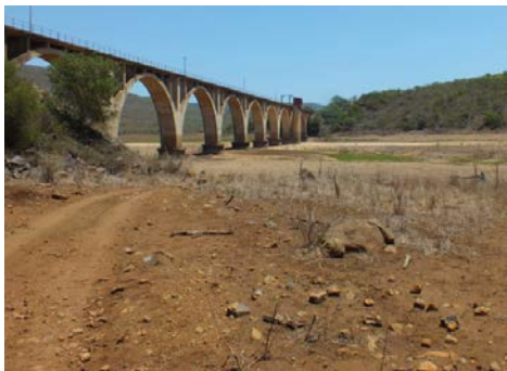
Figure 9: Pongola River Railway Crossing Water Level in September 2015.
