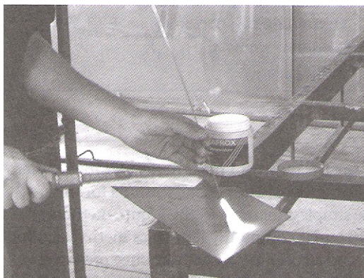
Figure 4.17: Welding with an oxy-acetylene torch
