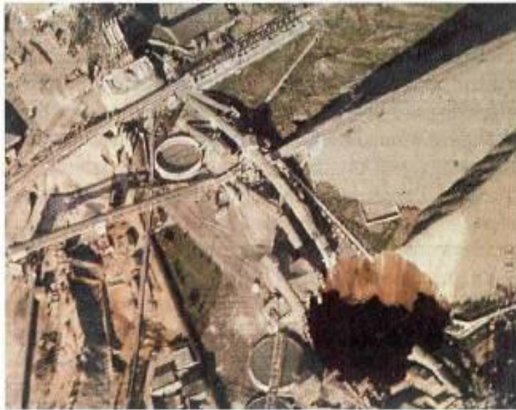
Plate 3 A sinkhole on a gold mine, which resulted in the deaths of 29 workers when a 3-storey crusher plant collapsed / fell down the hole (Swart et al. , 2003)
