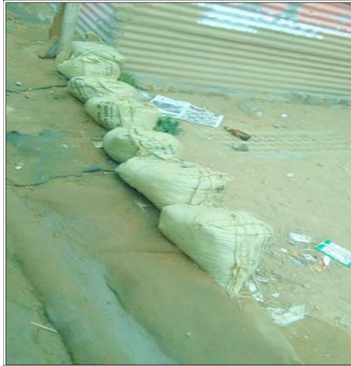
Figure 6.20: Mats used to absorb wastewater overflow in Section A
