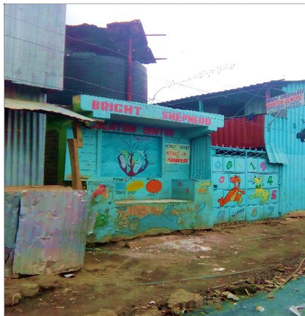
Figure 5.8: A water kiosk in Moto Moto village adapted into a kindergarten school
