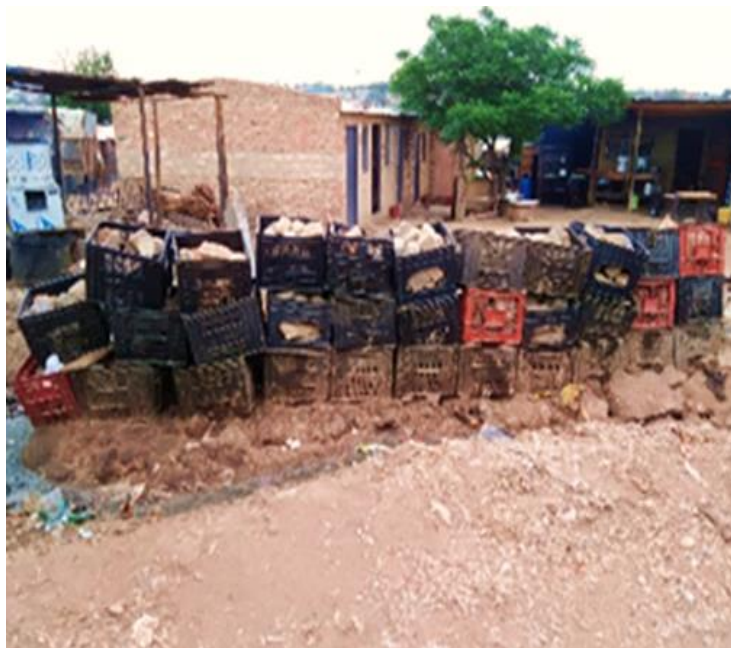
Figure 6.21: Plastic crates used to hold back floods and wastewater in Section A
