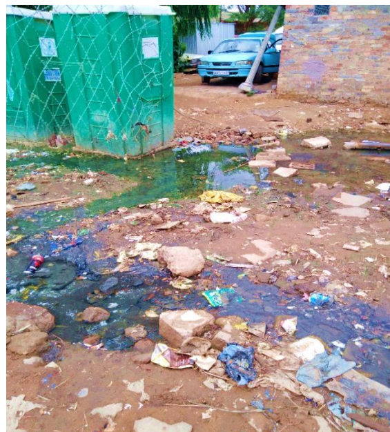
Figure 6.17: Poor waste-water disposal next to chemical toilets in Section D
