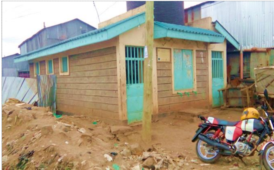
Figure 5.7: An abandoned ablution block in Riara village
