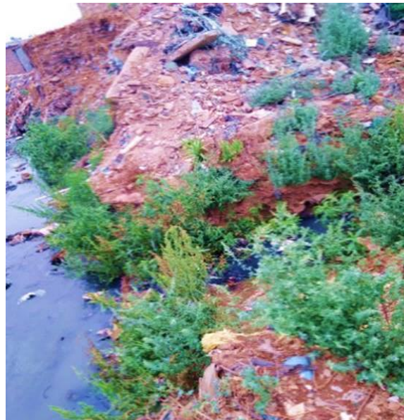
Figure 6.16: Jerry rigged wastewater tunnel emptying in Jukskei River in Section A
