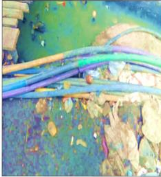
Figure 5.3: Color coding of pipes for identification by vendors
