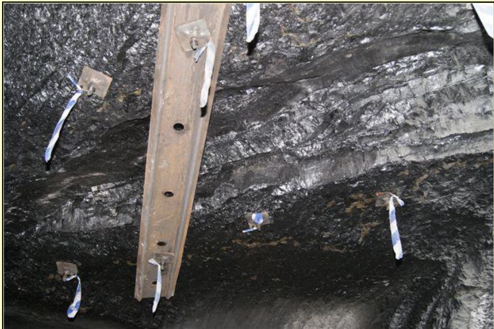
Figure 5-41 Picture of a dyke and the way it is being supported by W-straps and roof bolts at Boshmans shaft (X-Strata Coal)
