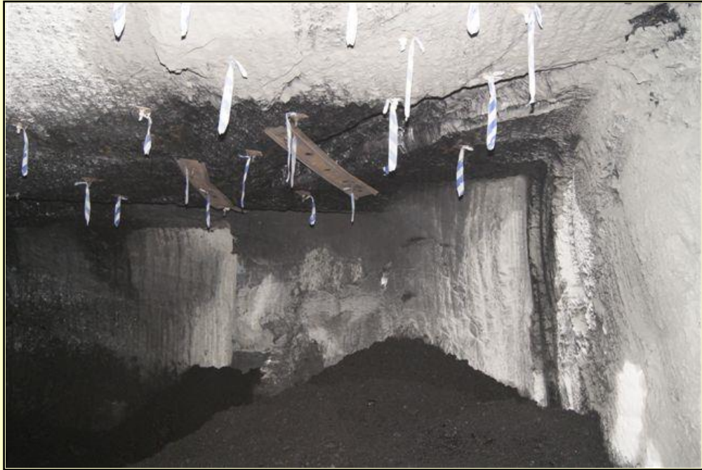
Figure 5-42 Picture of a coal face and the roof in the vicinity of a dyke at Boshmans Shaft (X-strata Coal)
