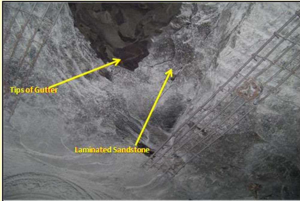
Figure 5-37 Picture showing the tip of guttering in a laminated Sandstone roof which is being re-supported by straps and roof bolts
