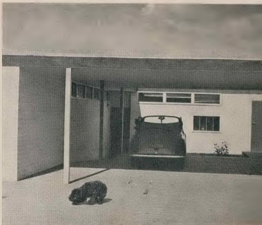
View of car port from road with main entrance on the left and the service door on the right.
