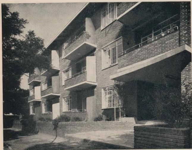
Below: View of flats from the street looking east.
