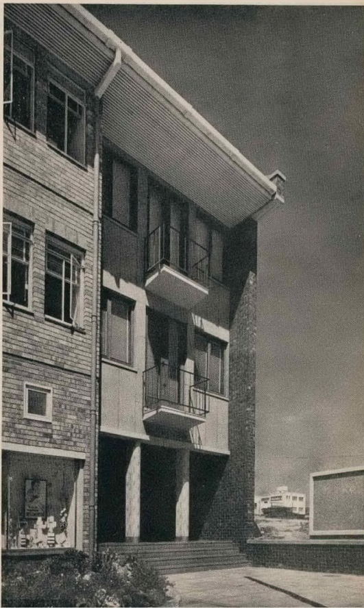
View showing detail of approach to main entrance.
