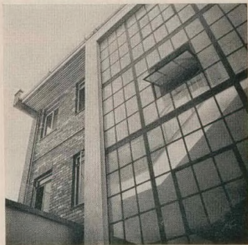
Below: Detail of staircase window facing court.
