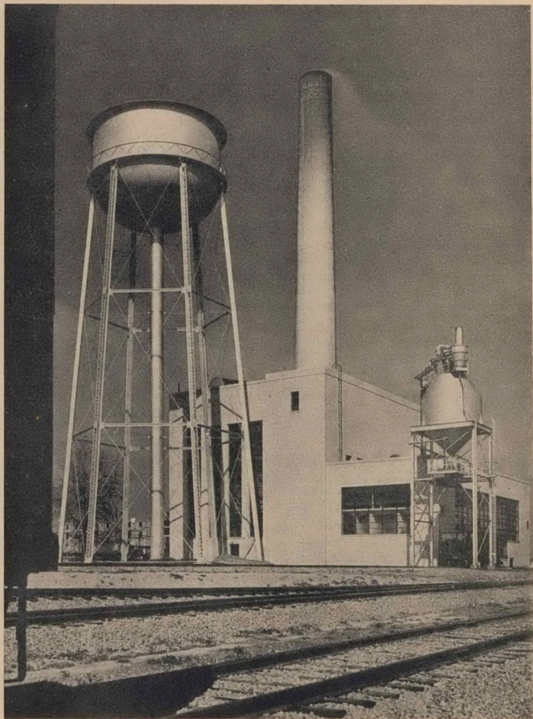
POWER HOUSE, CHEVROLET MOTOR AND AXLE DIVISION, TONAWANDA, N.Y.
