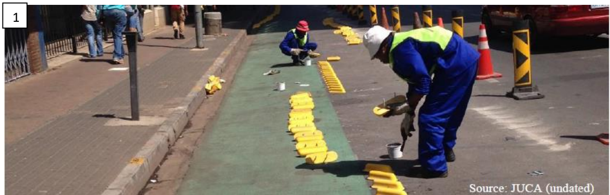
Figure 44: Construction of bicycle lanes in Braamfontein.
