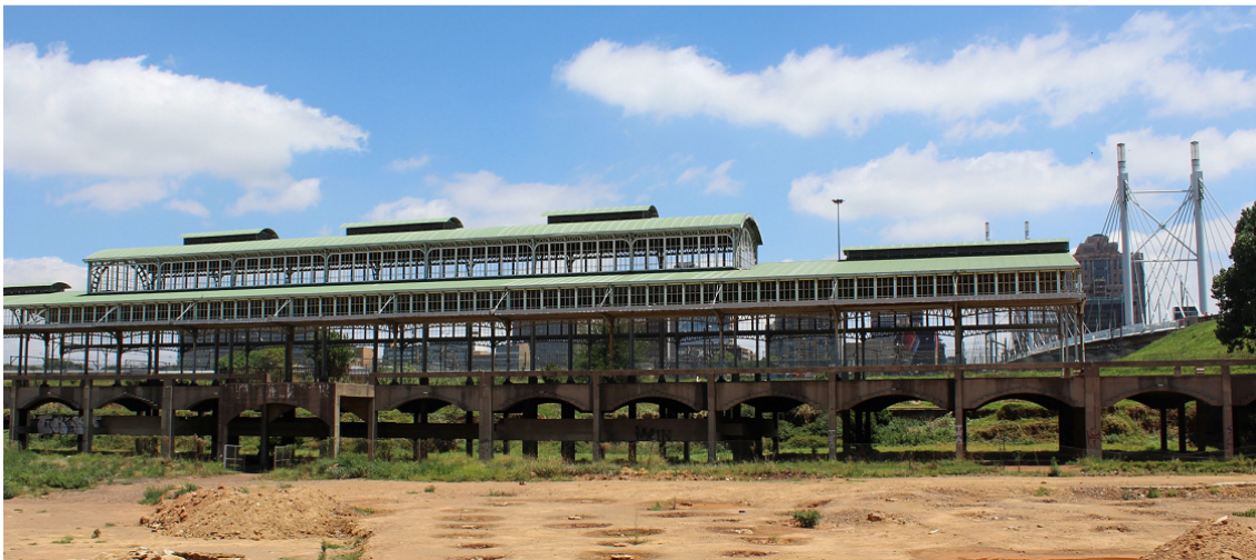
Figure 18: The old Park Station structure in its usual desolate state, with a glimpse of the Nelson Mandela Bridge on the right (author's photograph).
