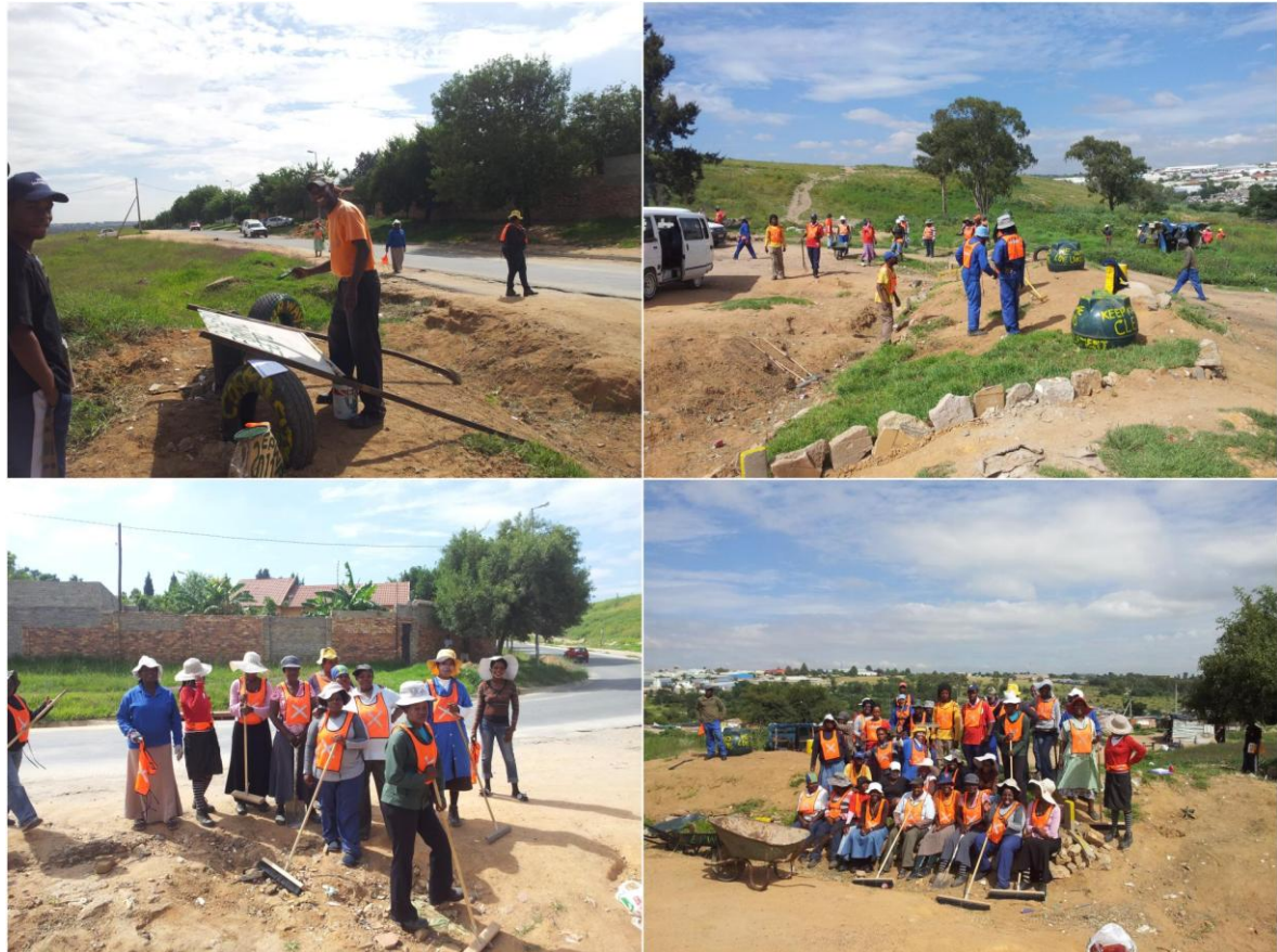
Figure 56: Workers on the Expanded Public Works Programme cleaning initiative cleaning and preparing a park at the entrance to the settlement on Agnes Ave
