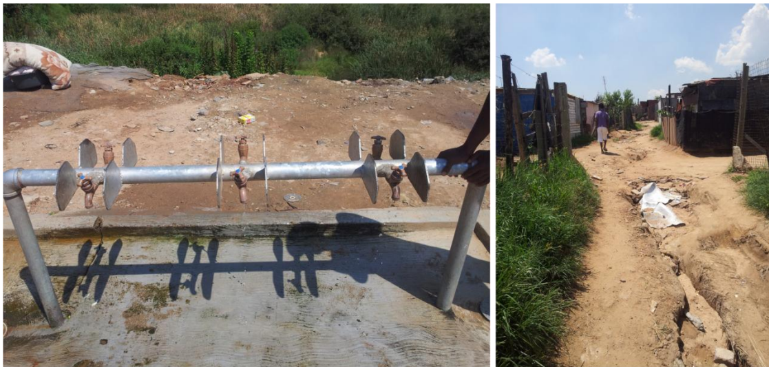
Figure 20: A Typical Standpipe and eroded roads due to lack of drainage systems in Kya Sands Informal Settlement
