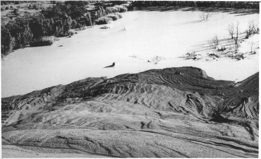
Figure 8.11 Failure of Sache's Dam East from the top of the dam wall, showing the transverse failure lines at right-angles to the wall.
