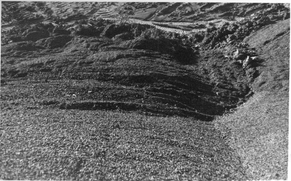
Figure 8.20 Failure of small dump on slime in pond of Sache's Dam West. Upper photograph shows slide taking place. Bottom photograph taken from the top of the small dump, shows the ridges of failure.
