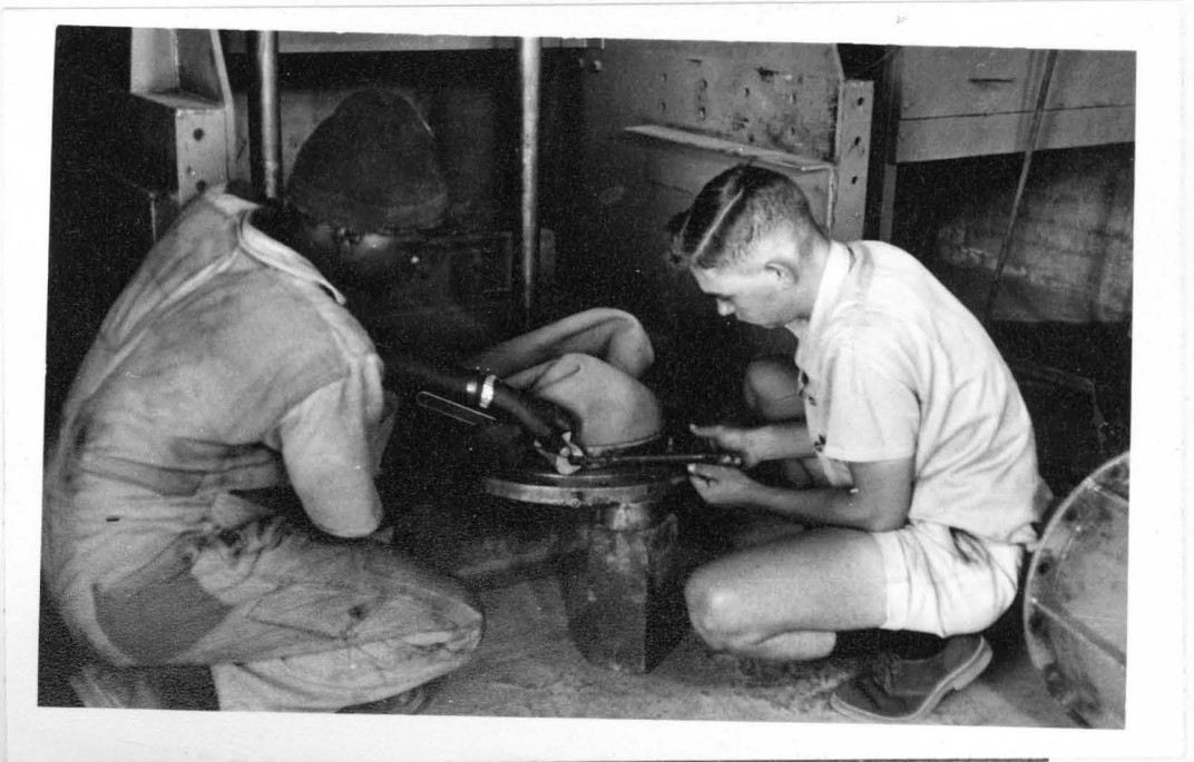
Figure 9.12(c) Strap around rubber rings tightened.
