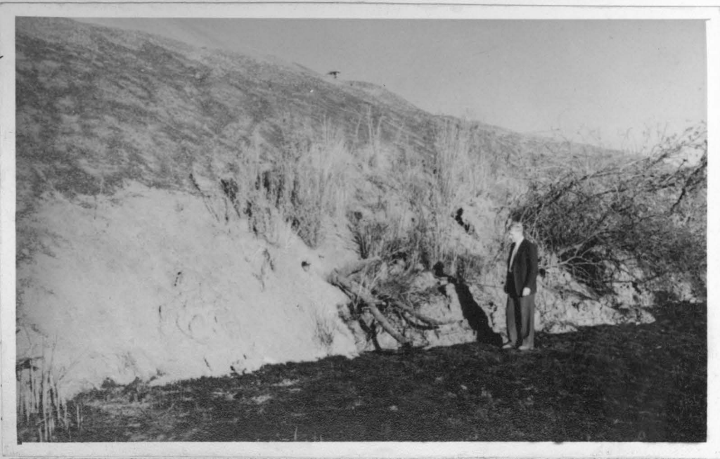
Figure 8.15 Dump No.3. Toe of slide uprooting trees.
