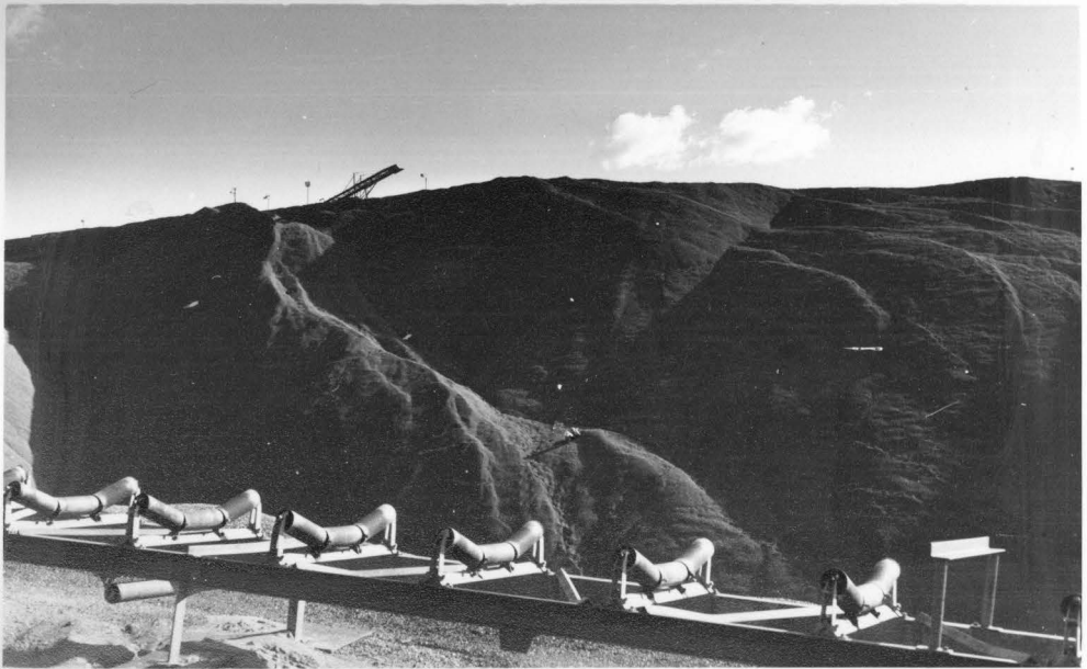
Figure 8.17 Failure of dump No.3. Back leg of failure. Photographs taken from Sache's Dam East wall.
