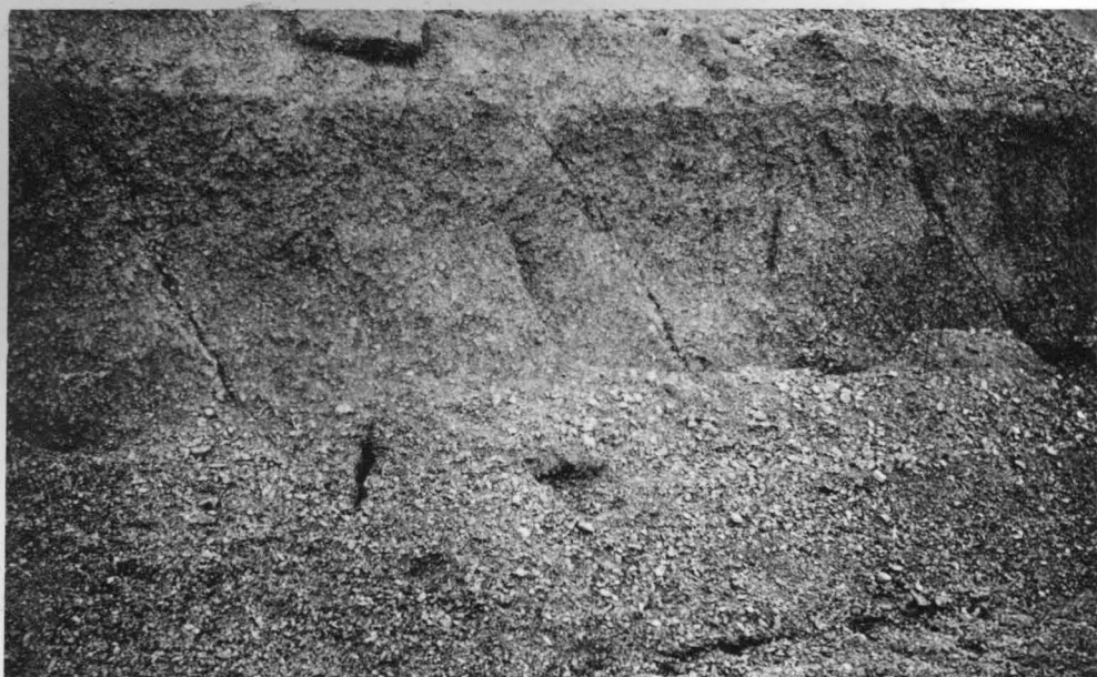
Looking east. Failure lines near left -hand side of failure on Figure 8.11. Note slope to the right.
