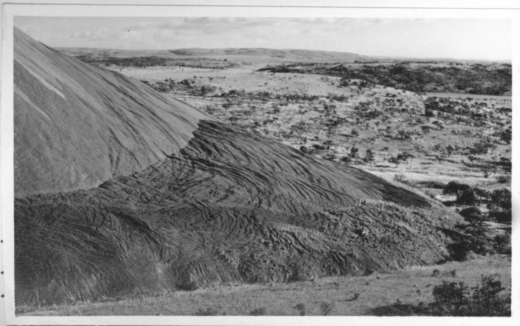
Figure 8.14 Failure of dump No.3 showing sliding failure. Note the old dump material (covered in grass) being pushed ahead.
