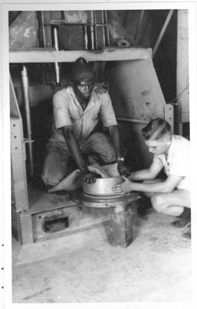
Figure 12(b) Rubber membrane slipped on to bottom bearing plate and rubber rings rolled on.
