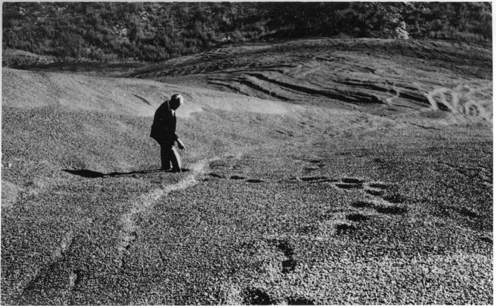
Close-up of failure at front leg of wedge.
