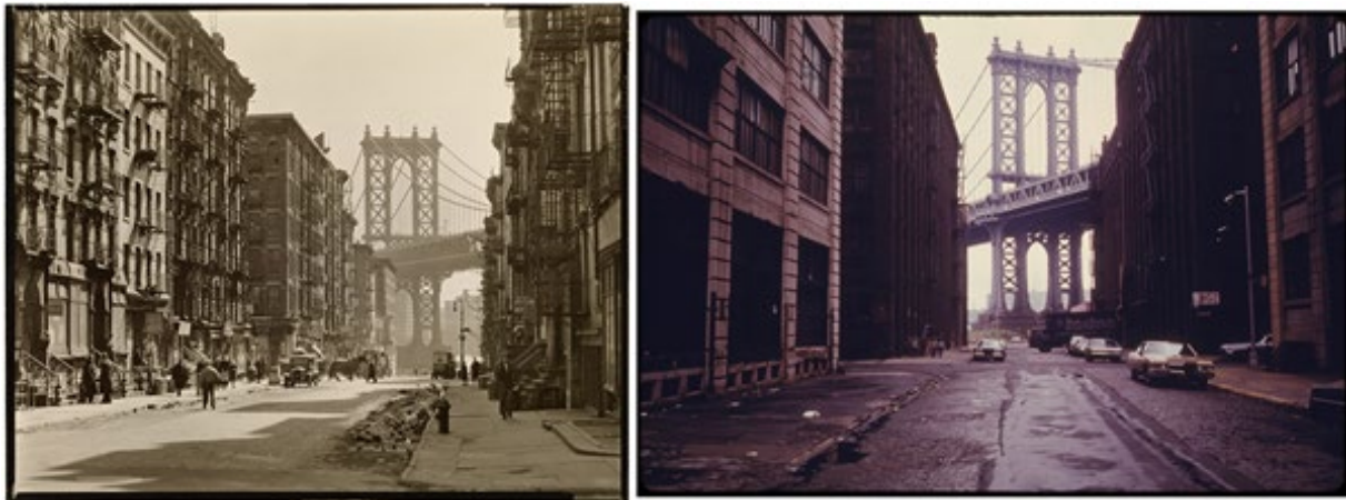
FIGURE 3.12. A side-by-side comparison of the two images of the Manhattan Bridge used in Polonia . The image on the left is of Pike and Henry Streets in Manhattan, 1936. The second, on the right, is from 1974, Brooklyn.
