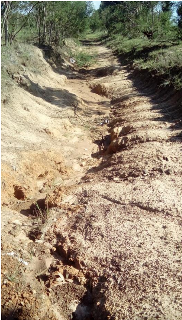
Figure A5 showing a developing gully due to soil erosion in the area
