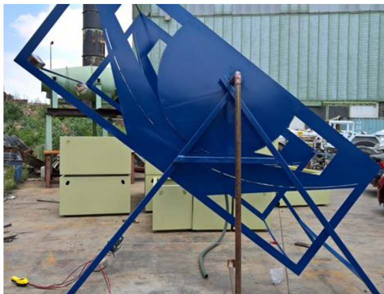
Figure D 3: Manually Testing Heliostat Winch Operation
