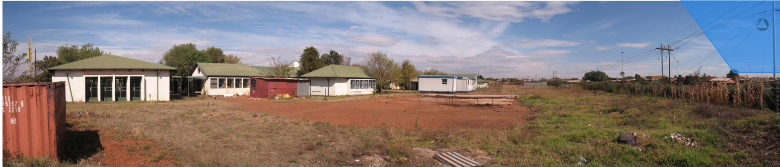
Figure 27 - Site photo with existing KRC buildings in the background (R.Hartmann).
