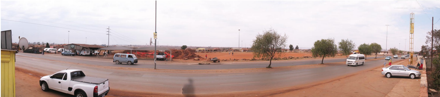
Figure 30 - Photo looking onto Maphike Street (R.Hartmann).
