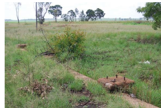
Figure 58. External wall foundations showing bolts for structural steel (Photo by G. Reeks)
