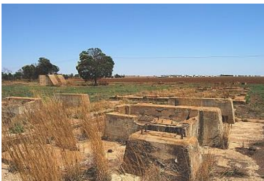
Part of the foundation complex of the secondary crushing plant
