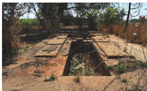
Figure 47. Foundations for two boilers
