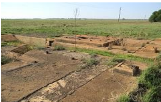
Motor and column foundations in receiving area jigs of secondary crusher
