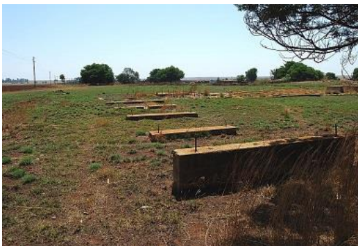
Line of trestles foundations for incline conveyor chute to crusher
