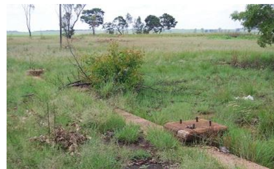
Column and wall foundations of the boiler house
