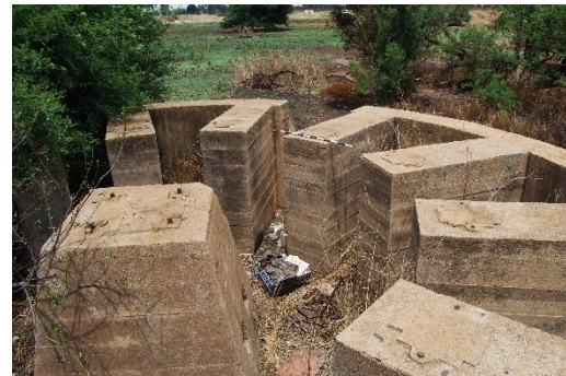
Figure 56. Foundation of part of the Godfrey roaster. (Photo by G. Reeks)
