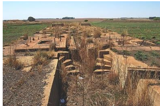
Complex concrete foundations in the secondary crushing area
