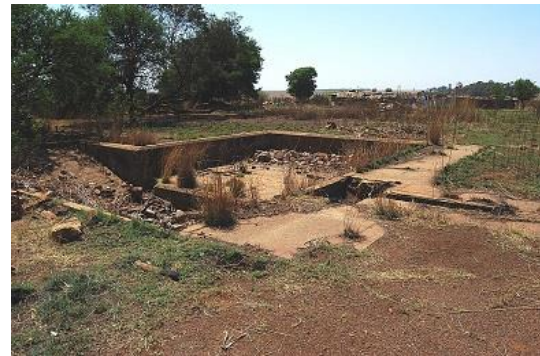
Part of the feeder station to the roasting plant
