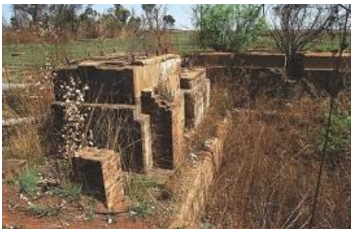
Generator foundation inside the boiler house foundations
