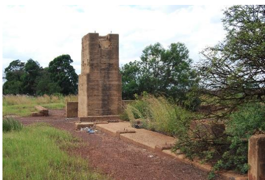
Figure 45. Foundations of the Roasting plant 2016. (G. Reeks Photo)
