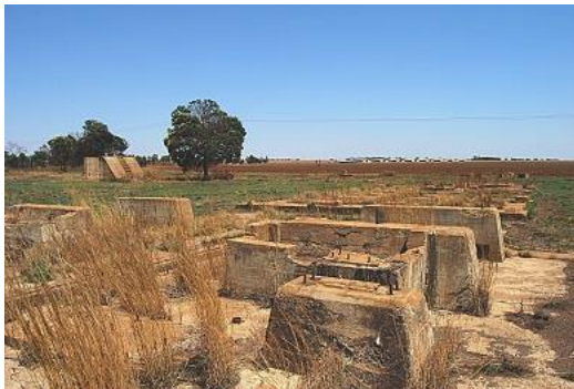
Foundation plinths of the Hardinge Ball Mill machines
