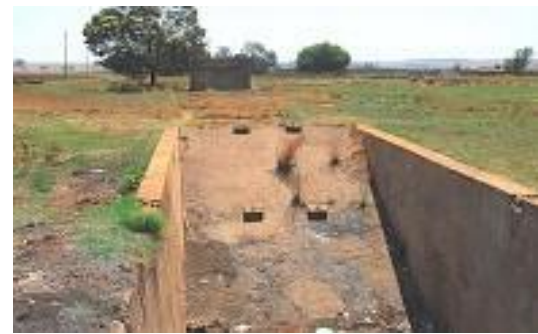
Discharge end with foundations for trestles of conveyor
