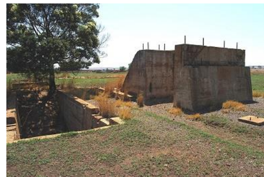
Very large foundation blocks and incline ore of the primary crusher
