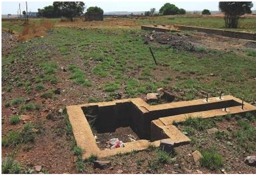
Foundation for manual rail points unit
