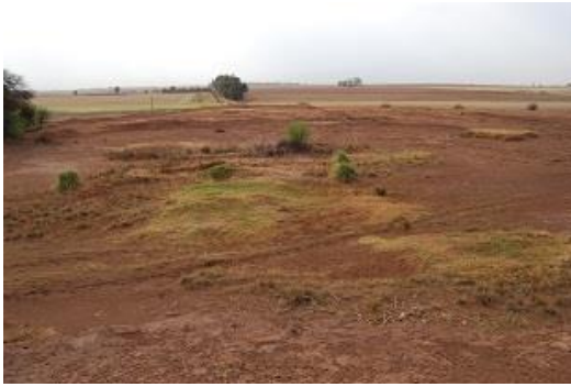
Slimes dam - top surface
