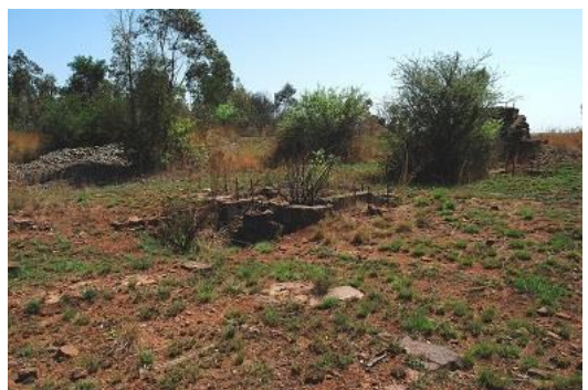
1890s motor or engine foundation for the Blake jaw crusher
