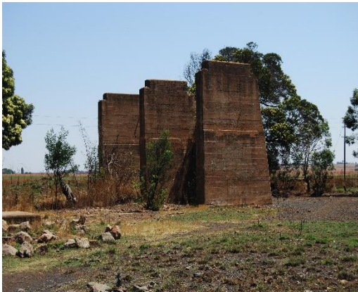
Figure 51. Foundations of the smelter furnace (Photo by G. Reeks)
