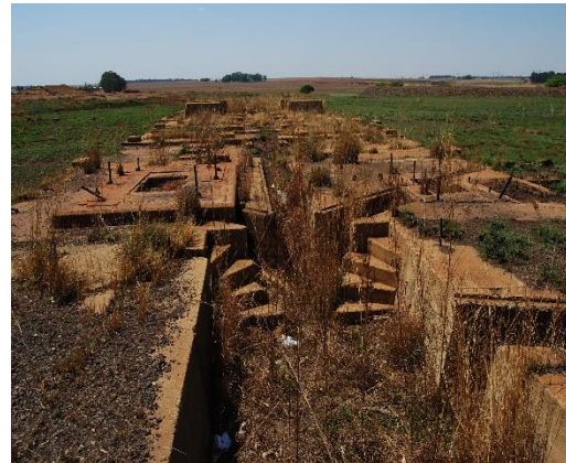
Figure 52. Foundations of the ball mills and the flotation plant. (Photo by G. Reeks)
