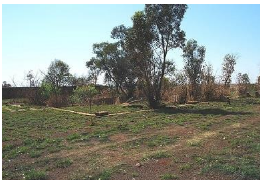
Wall and column foundations of boiler house
