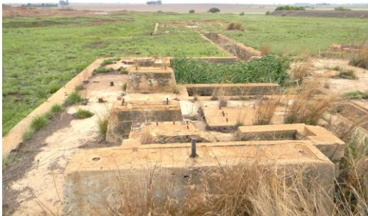
Door Rake classifier foundation area looking towards Flotation plant
