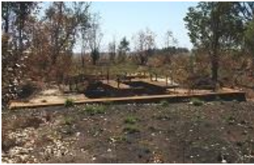
Foundations of the shaft head gear motors and winder
