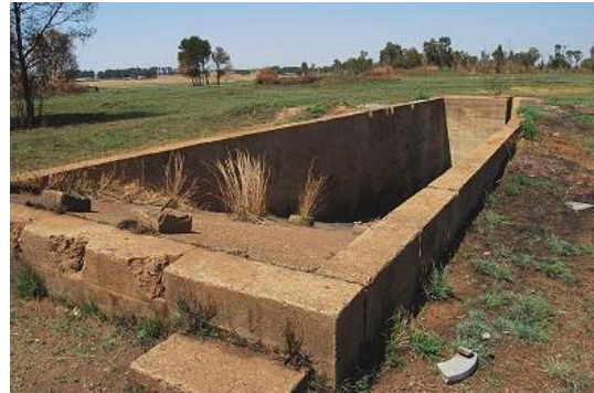
Ore chute to feed first conveyor to primary crusher plant
