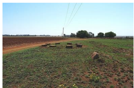
Foundations of the large water tower seen in figure 33
