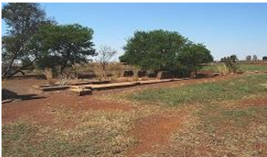
Feeder area foundations for the smelting plant
