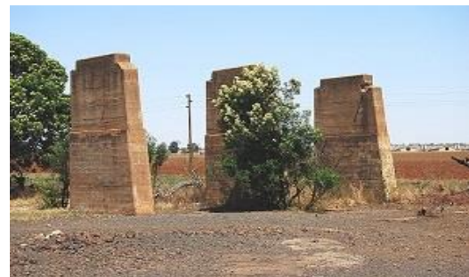
Support foundations for floors and smelting furnaces
