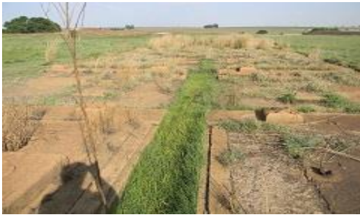
Harz jig foundations looking towards Hardinge Ball mill area
