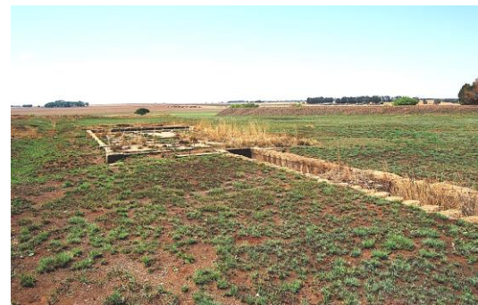
Large concrete trough feeding to MS Flotation plant foundations
