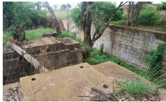
Boilers charge floor area
