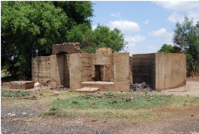
Figure 69. Concrete foundations for the Godfrey type Roaster at the TSBM mine. (G. Reeks photo).
