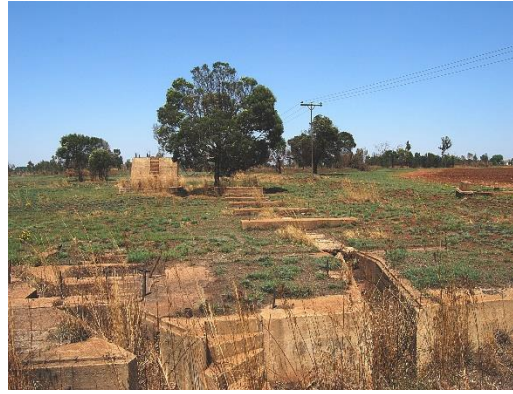
Figure 54. Foundations of the primary crusher plant. (Photo by G. Reeks)
