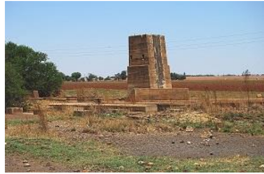
Concrete foundation for Huntington- Hubelein roasting pots
