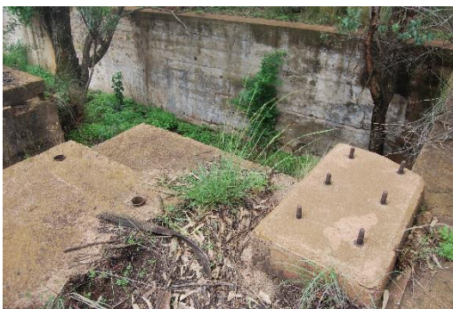
Figure 57. One of the foundations in the Boiler house showing machine bolts. (Photo by G. Reeks)
