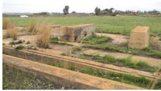
Concrete plinths for Hardinge Ball mill
