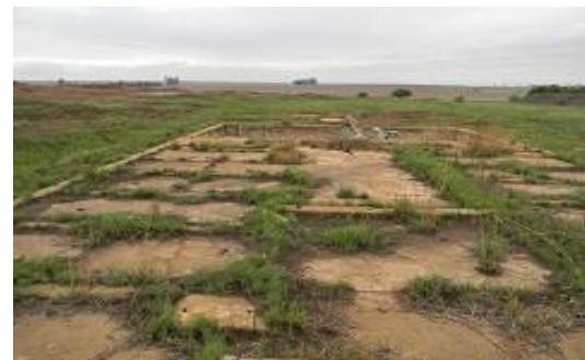
Foundations of two banks of 10 cell MS machines
