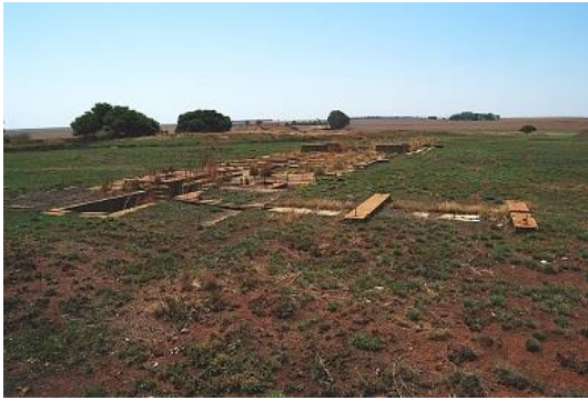
Initial feed area of secondary crushing plant crusher
