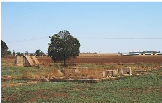
Wide view of the primary and secondary crushing plants
