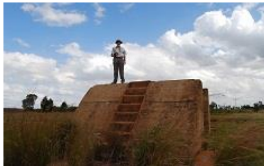
Foundation blocks of the primary crusher plant
