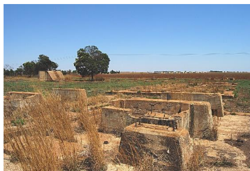
Figure 62. The plinth supported the bearings of the Hardinge Conical ball mill. (G Reeks photo)
