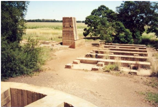
Figure 55. Foundations for roaster station. (Photo by G. Reeks)
