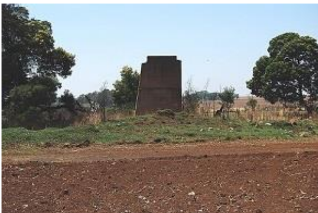
Support foundation looking from where the inclined feed conveyor would have been. The grassy mound has three concrete foundations in it which supported the trestles for the conveyor seen in Figure 42. Note the lumps of white limestone present on the soil in the foreground.
