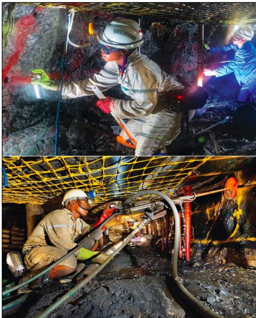
Figure 23: Marking and Drilling of an Underground Stope (Minerals Council South Africa, 2019j)
