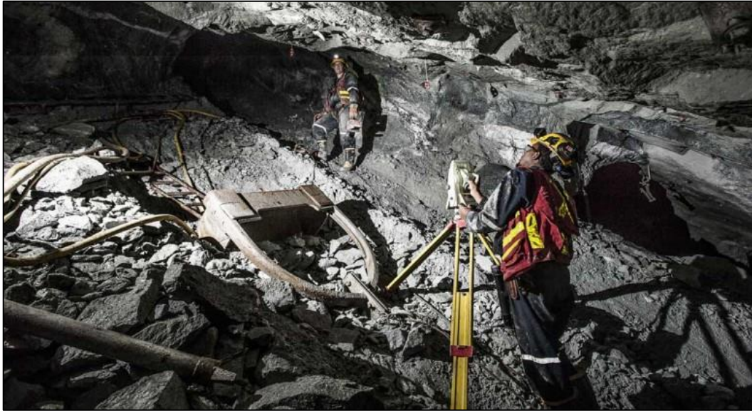
Figure 30: Underground Surveying (Tarikh, 2016)
