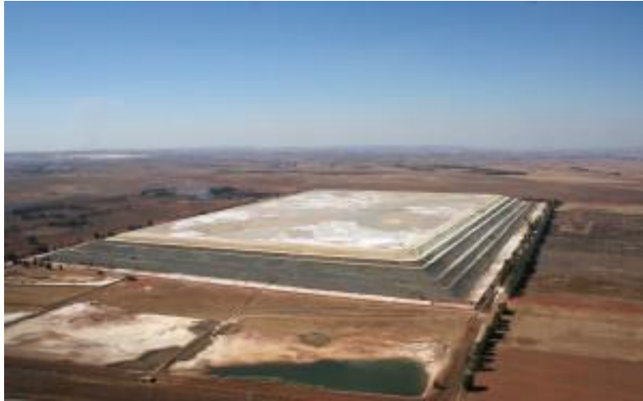
Figure 8: An aerial view of the Cooke tailings dam (MiningNews, 2013)
