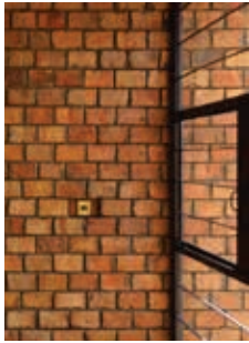
Clockwise From Top: Fig 4.25: Interior view Dorm Room; Fig 4.26: Exterior meeting Space; Fig 4.27: Lecture space; Fig 4.28: Brick and Window Detail; Photo Credit: Divisare.com
